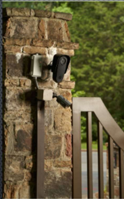
Electric & Existing Structure / Pole
