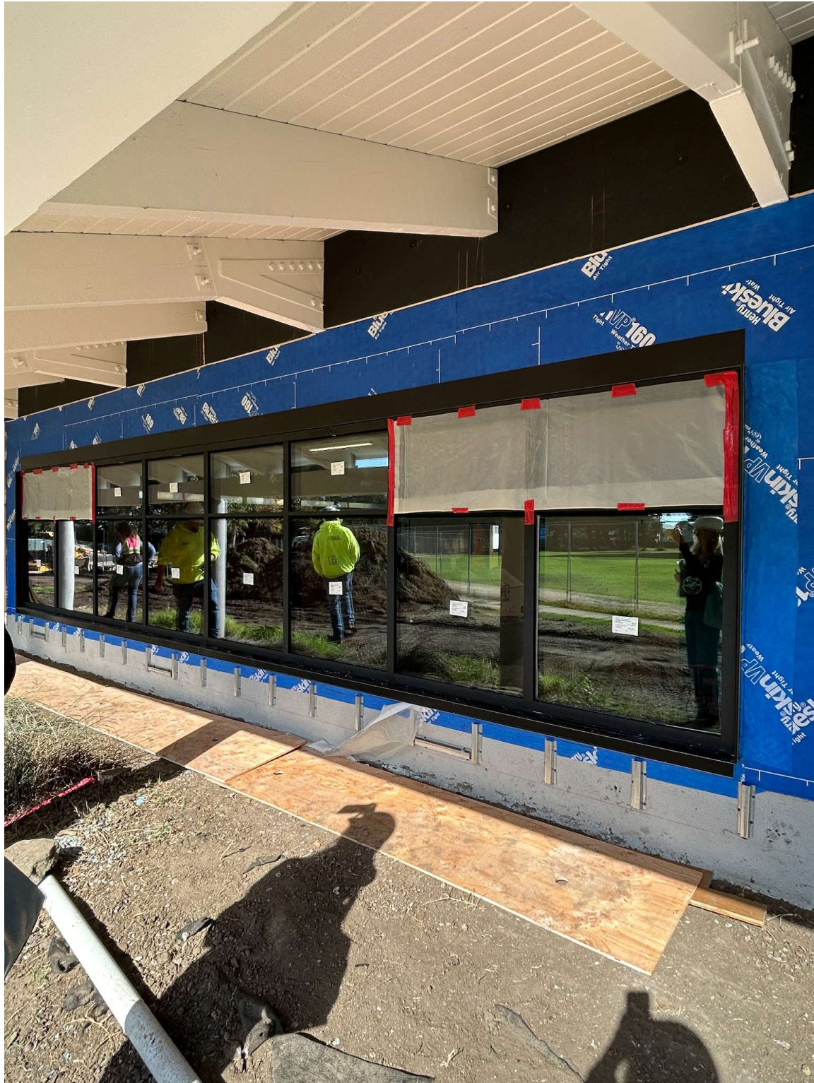
Installation of new storefront system with weatherproofing membrane and flashing
