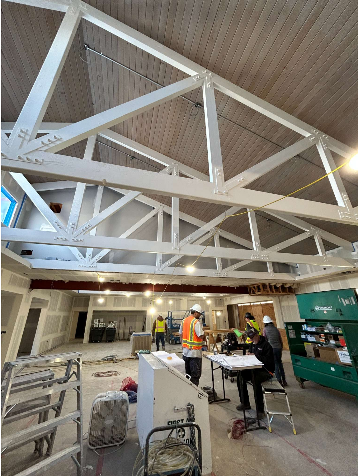
Exposed truss system fully painted
