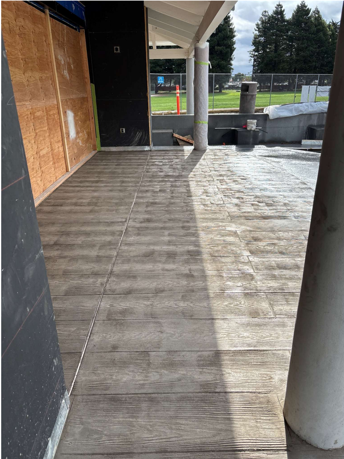
Decorative concrete patio slab placed and stamped with wood-plank pattern
