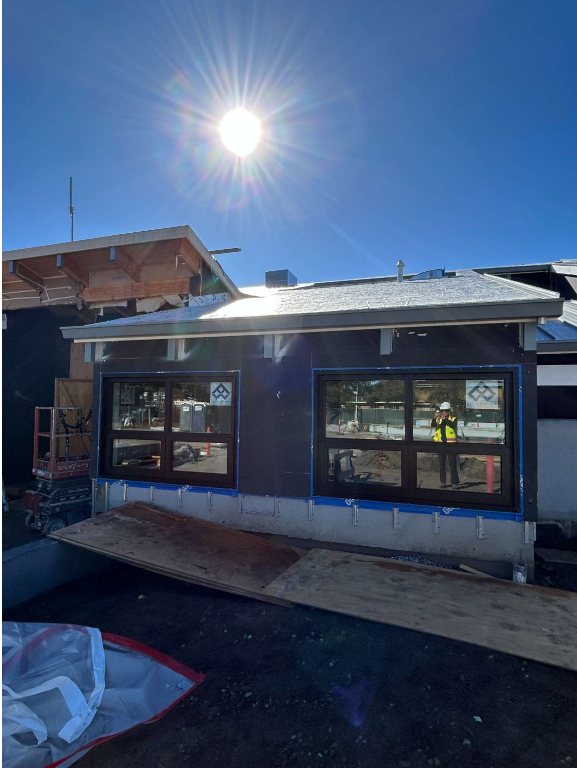
Front office window units installed, surrounded by exterior sheathing and waterproofing
