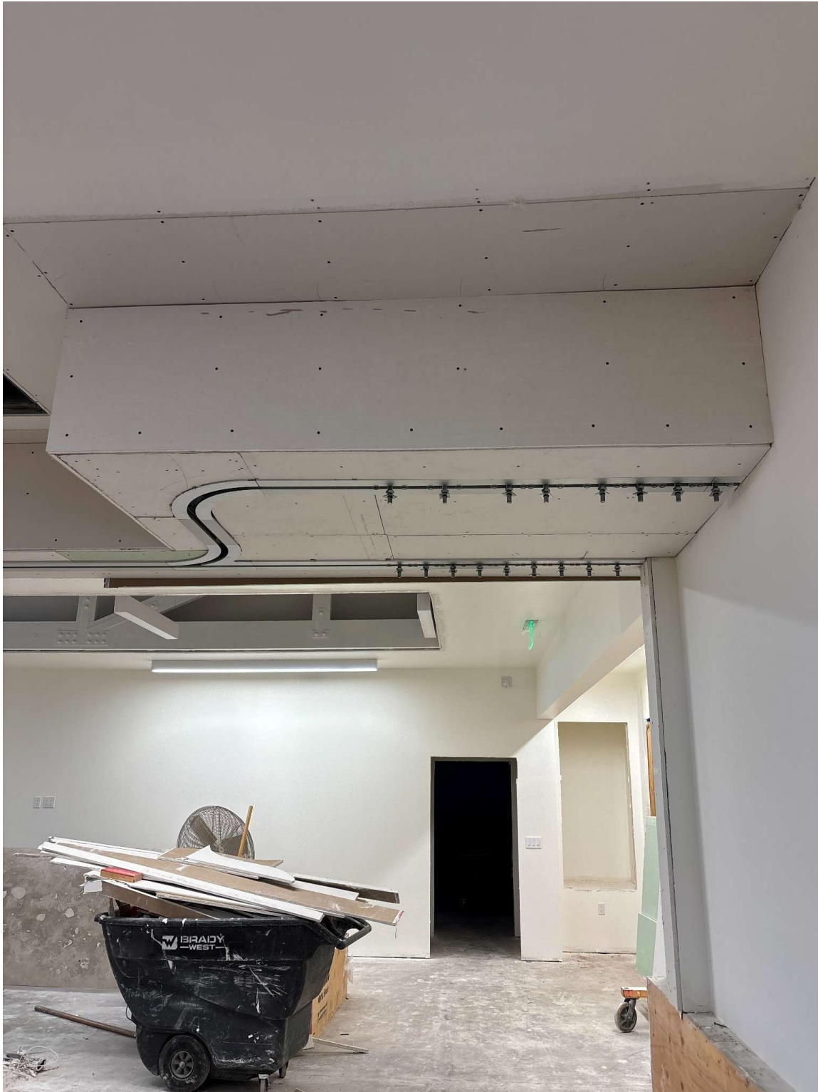
Interior soffit framing and drywall enclosure to house the operable partition track system
