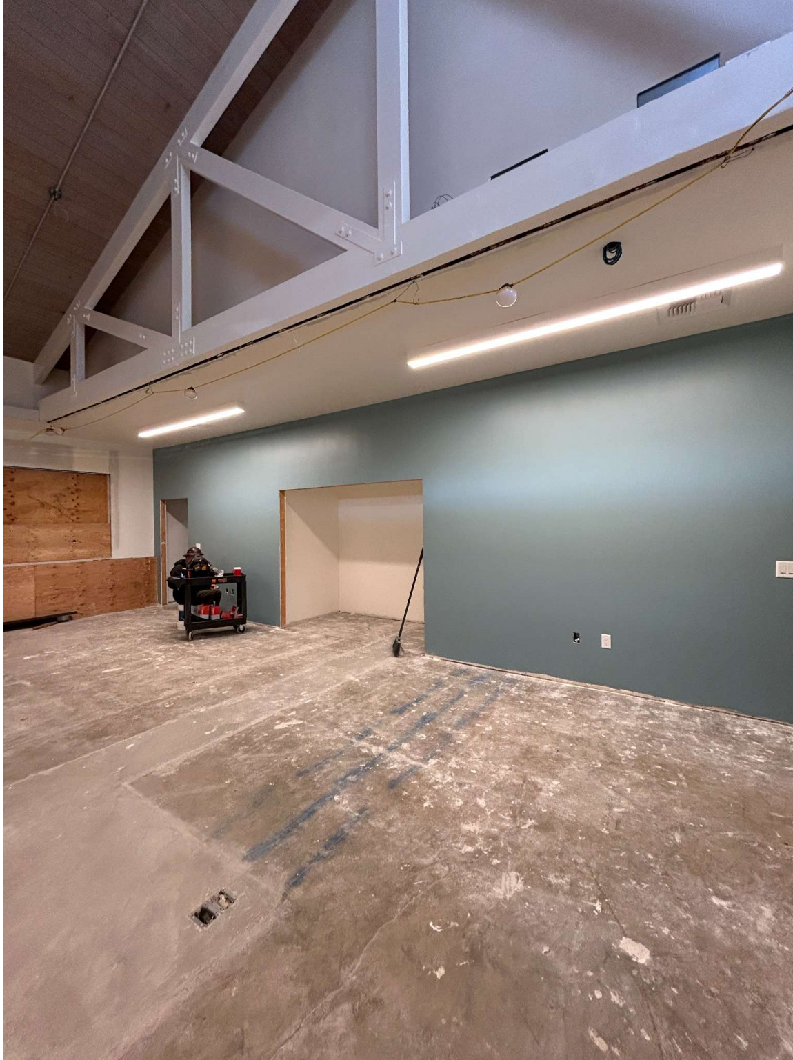
Interior progress with wall paint applied and linear LED lighting
