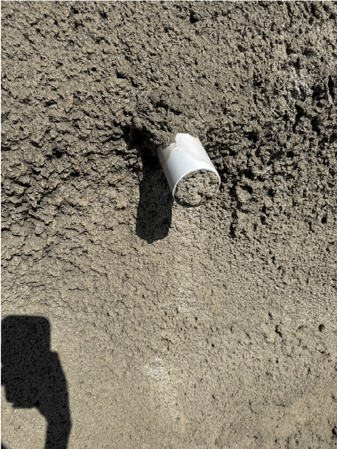
Photo 6: Closeup of a shotcrete plugged weephole - 2 April 2025
