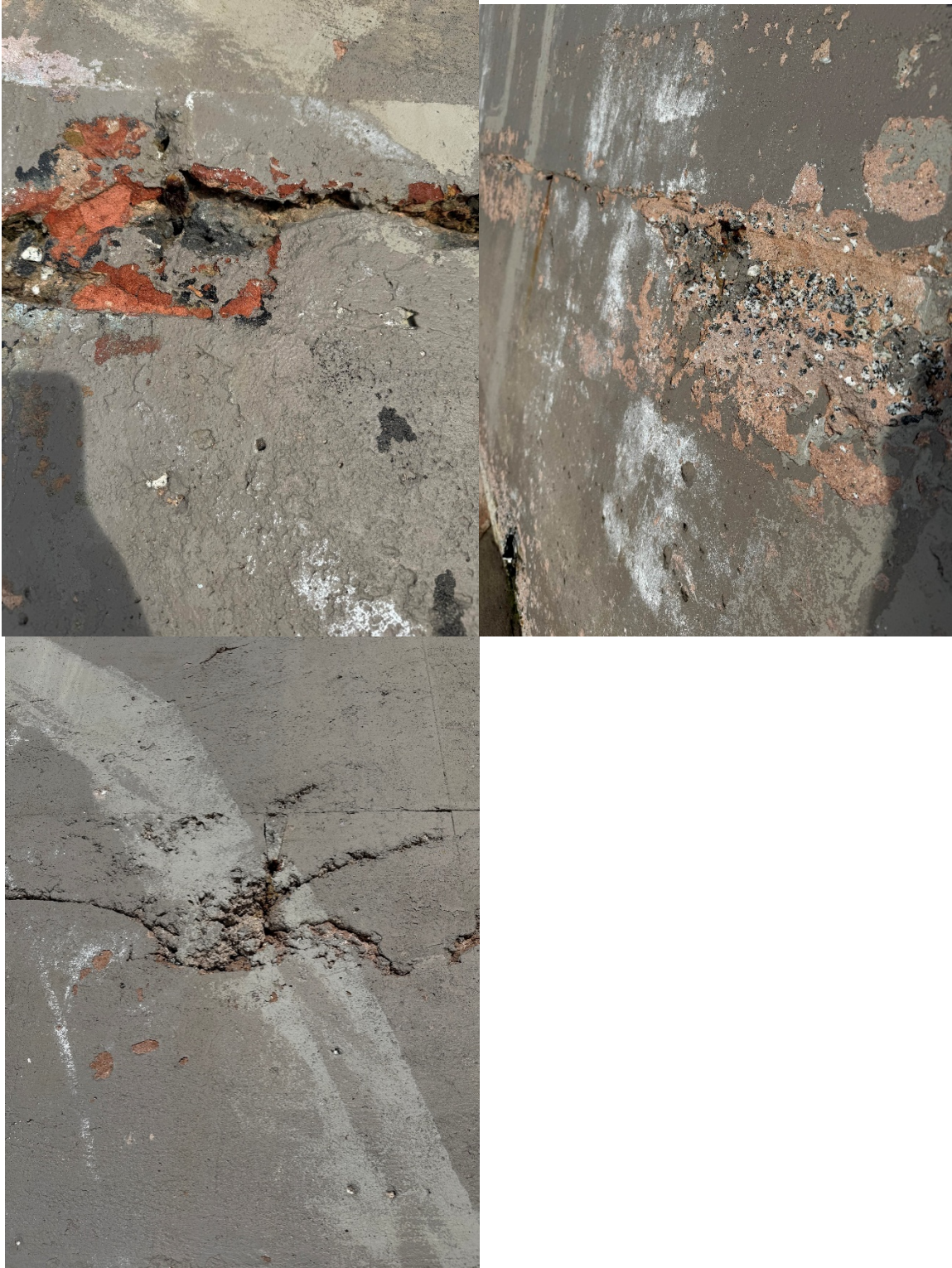
Photo 9: Concrete Spalling of Gravity Seawall, Typical - 2 April 2025
