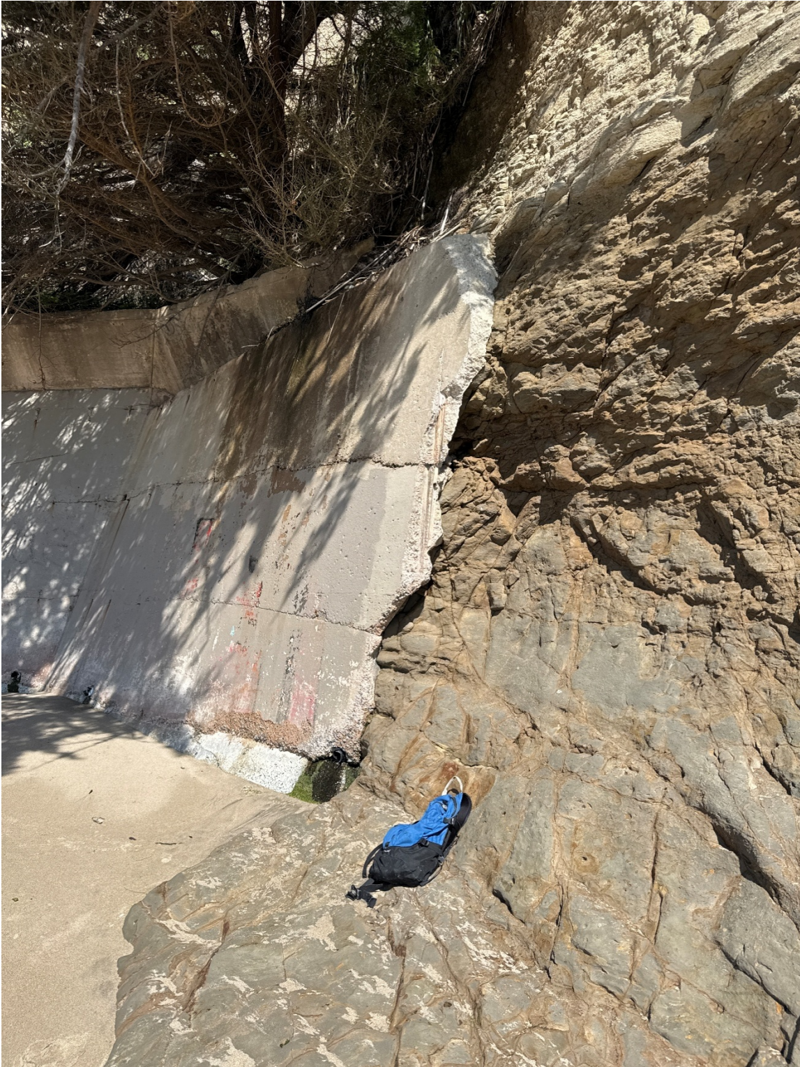
Photo 8: Minor Outflanking of Gravity Seawall at 4820 Opal Cliff - 2 April 2025
