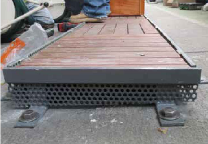
Perforated steel perimeter between platform and street to allow stormwater to flow from crown to gutter
