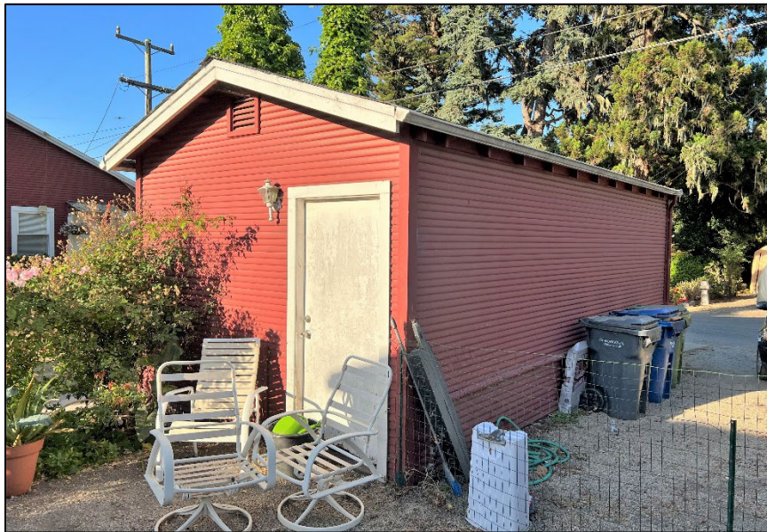
Photograph 7: Garage viewed from the north corner, showing secondary entrance on the northeast gable end of the building and lack of fenestration on the northwest side. Camera facing south, June 22, 2022.
