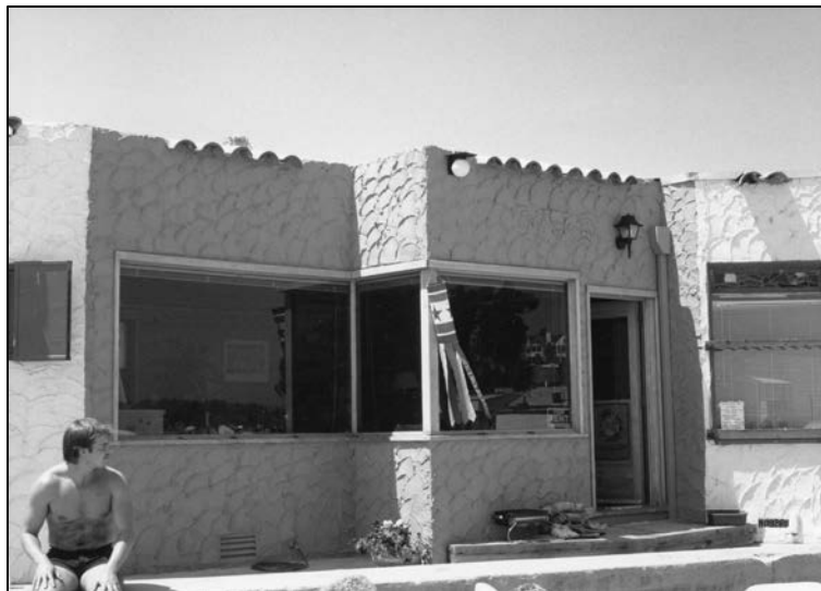
Figures 6 and 7. Top image is a circa-1950s image of the subject unit. Bottom image is taken from the 1987 National Register Registration Form. Note the conversion of a window to a front (south) elevation door and enlargement of window openings in the subject unit ( Courtesy: City of Capitola Planning Department ).
