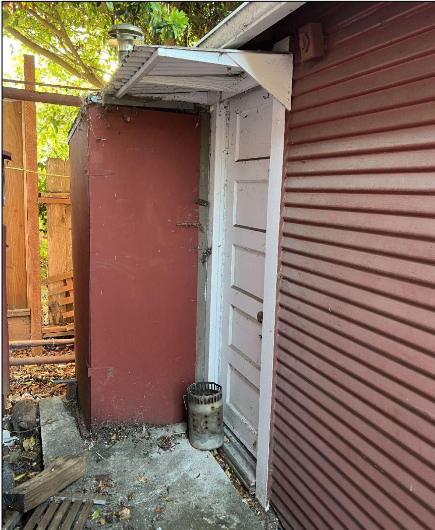
Photograph 11: Detail view of the paneled wood door at the secondary entrance to the storage building. Camera facing south, June 22, 2022.
