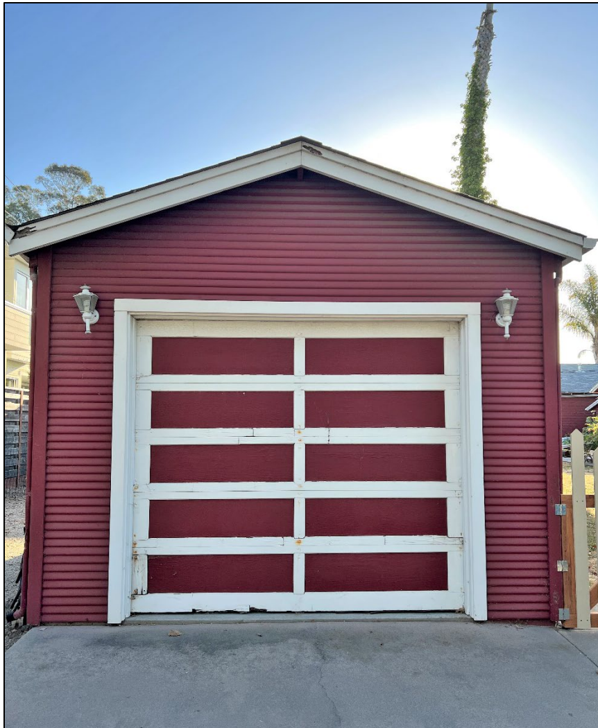
Photograph 6: Southwest façade of the garage, showing tilt-up, paneled wood door. Camera facing northeast, June 22, 2022.
