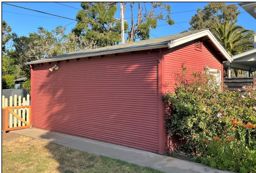
Photograph 8: Garage viewed from the east corner, showing lack of fenestration and ornamentation on the southeast side. Camera facing west, June 22, 2022.
