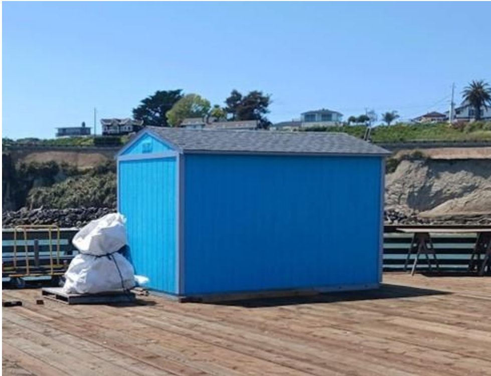
Figure 4. Existing Storage Shed (above)
