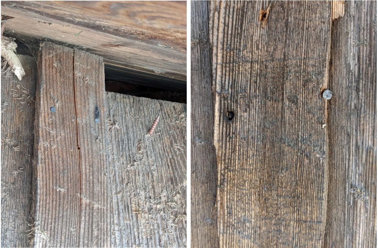
Detached Garage Round Nail Examples – Details, August 2022 (Photo by Leslie Dill)
