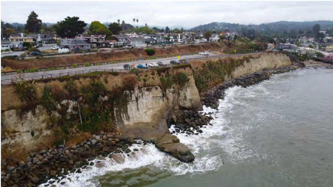
Photo 1: Existing view of the bluff
