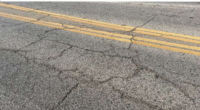
Alligator Cracking
