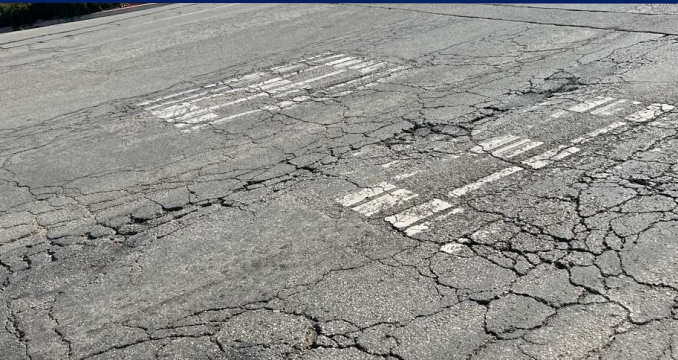
Depressions and Uneven Pavement
