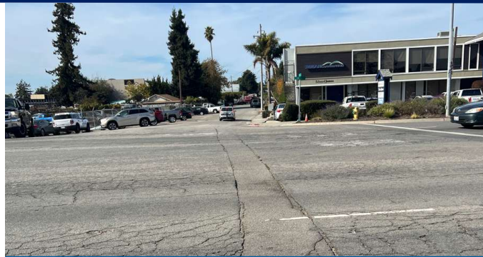
Old Utility Trench Repairs and Faded Striping
