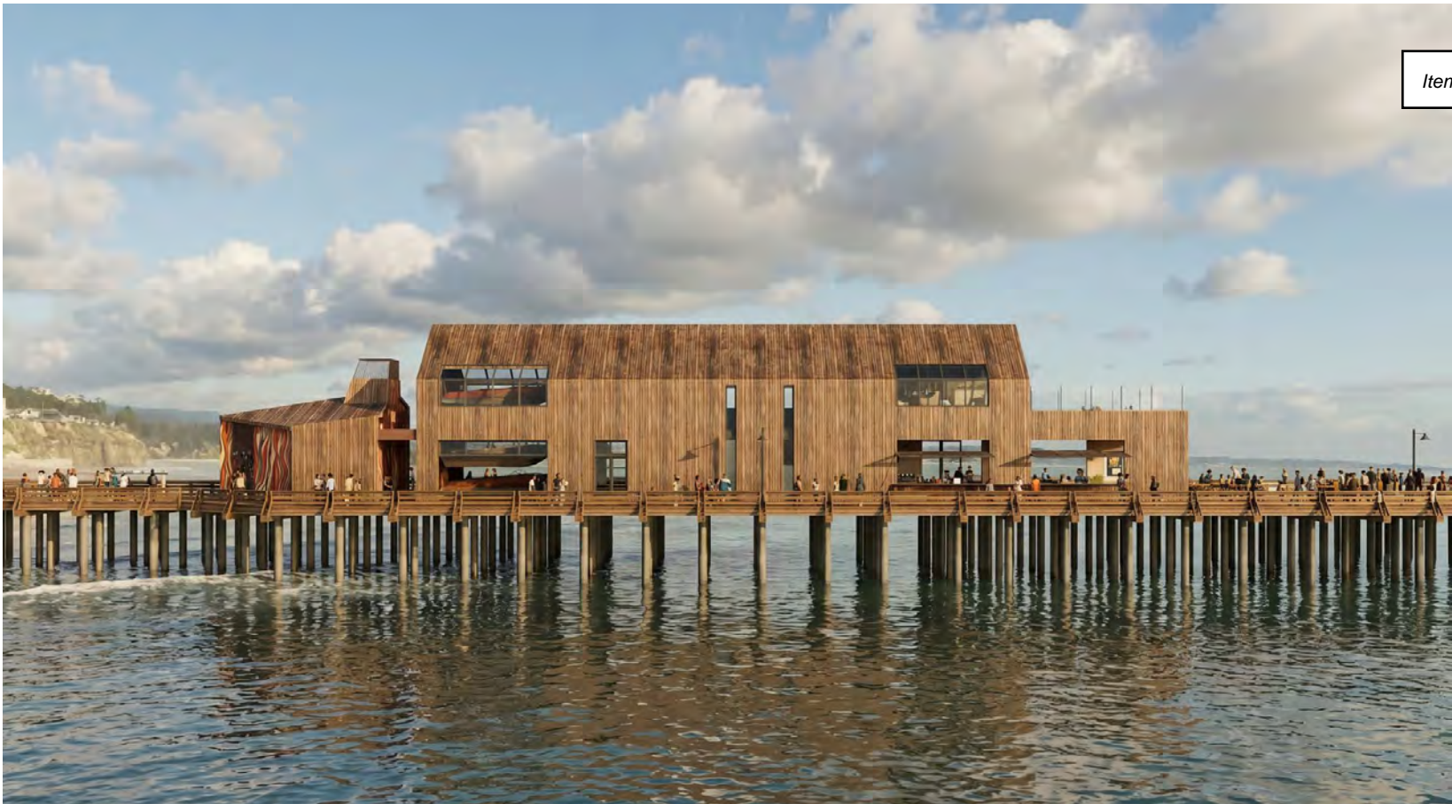
SIDE OF WHARF HOUSE & BOAT/BAIT HOUSE - VIEWED FROM CLIFF / MID-DAY
