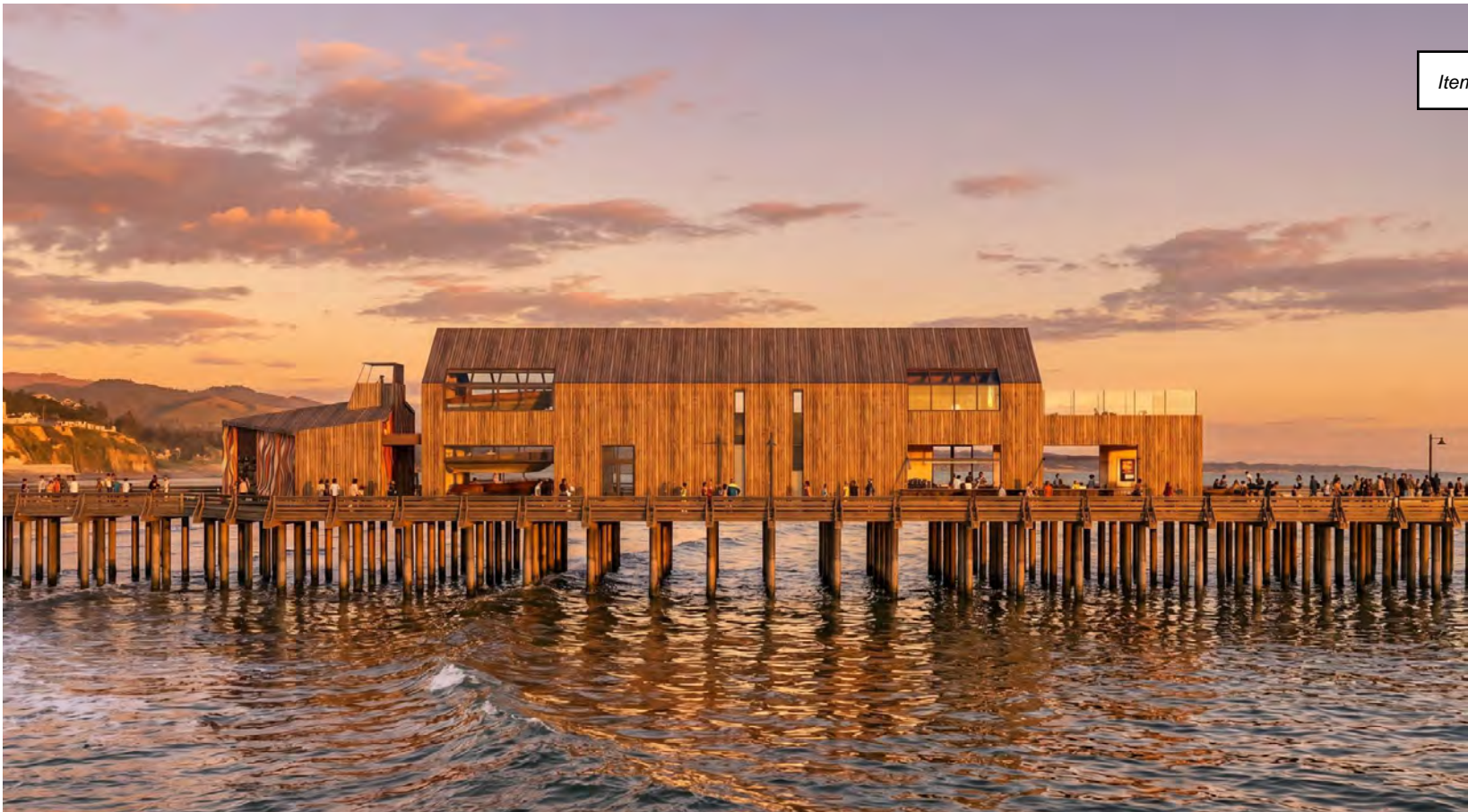
SIDE OF WHARF HOUSE & BOAT HOUSE - VIEWED FROM CLIFF / SUNSET
