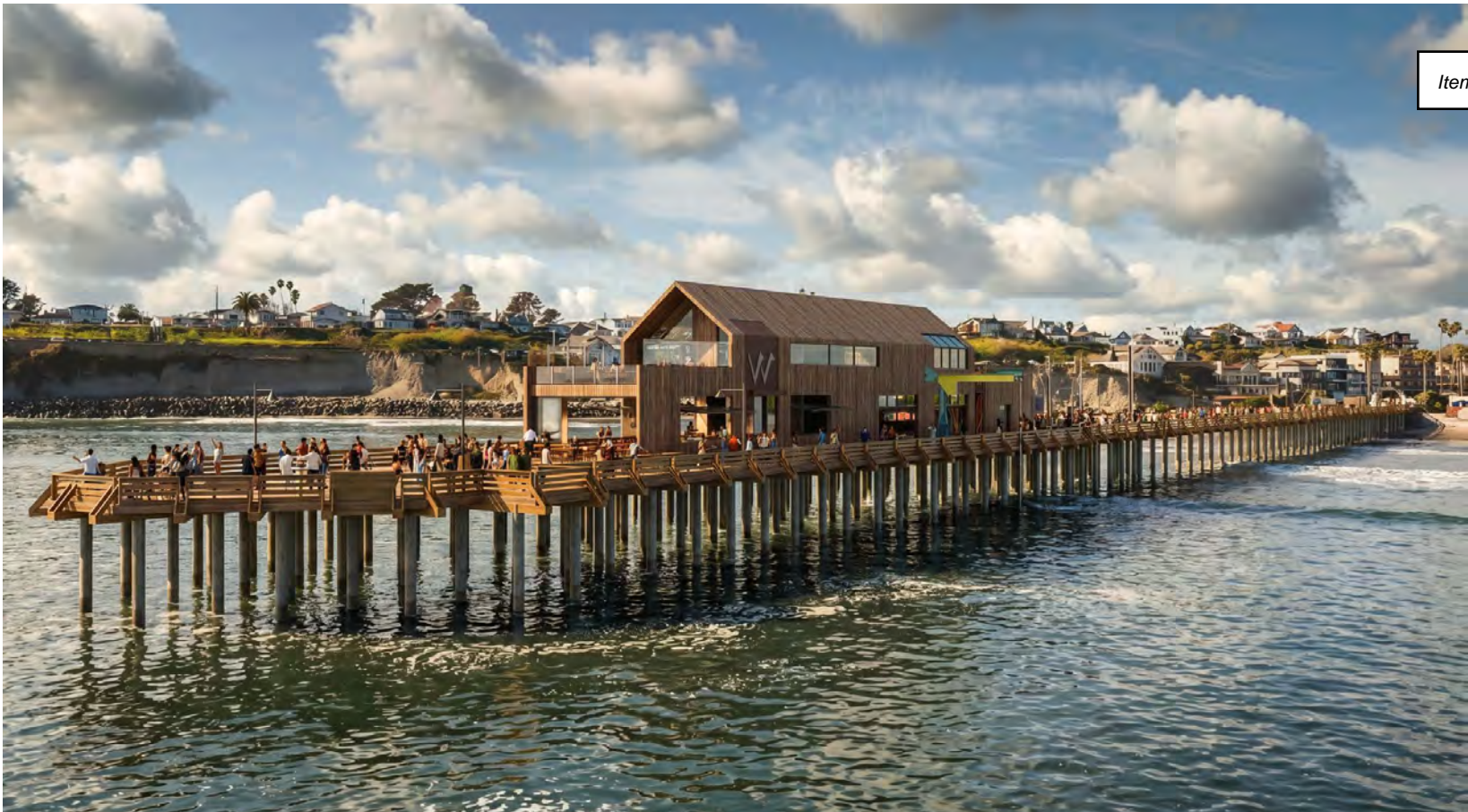
FRONT SIDE OF WHARF HOUSE / MID-DAY
