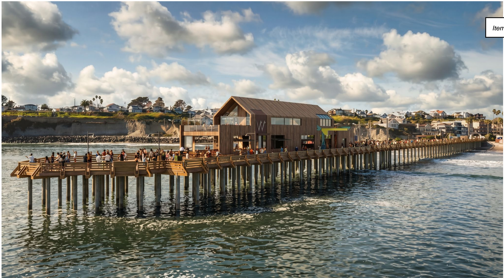
FRONT SIDE OF WHARF HOUSE / MID-DAY
