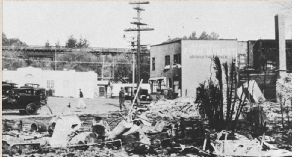
The surviving building was the Canepa Capitola Fish Market
