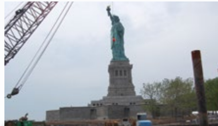
Liberty Island Installation Site
