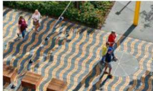
SPECIAL PAVING EXAMPLE - CURVED UNIT PAVERS
