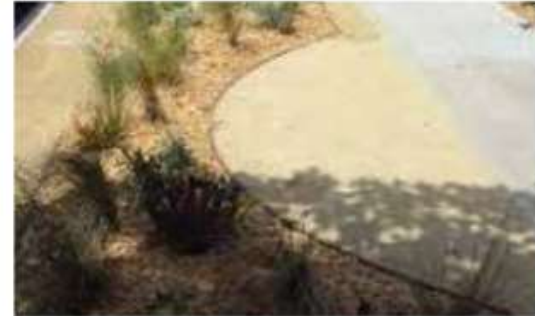
DG SHOULDER ALONG SIDEWALK
