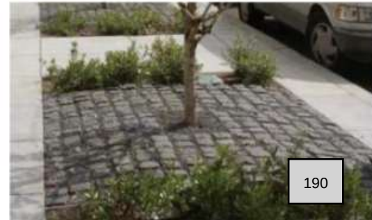
PERMEABLE PAVERS AROUND STREET TREES
