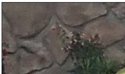
<E> STONE VENEER TO BE MATCHED OR REPLACED PER CLIENT CHOICE
