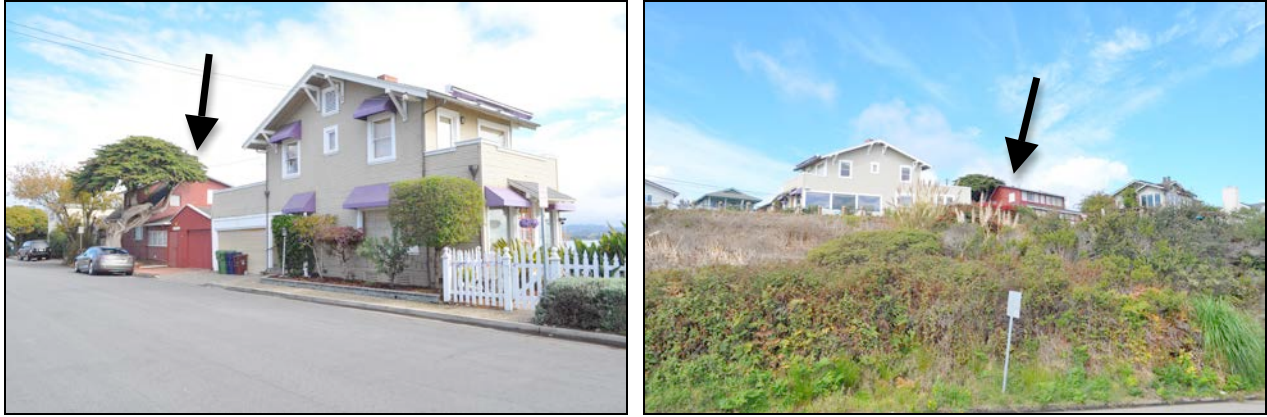
Figures 5 and 6. Left image shows the rhythm of gable roofs and false front roofs along Prospect Avenue, looking north, with the subject property indicated by an arrow. Right image views the variety of historic rooflines along the ridge looking northwest from Cliff Drive.
