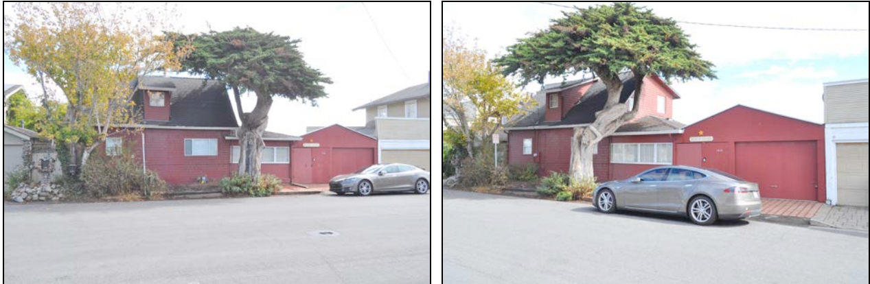
Figures 1 and 2. Left image shows the Prospect Avenue (west) elevation, as viewed from the street. Right image details the west elevation, showing the false-front, gable-roofed garage.
