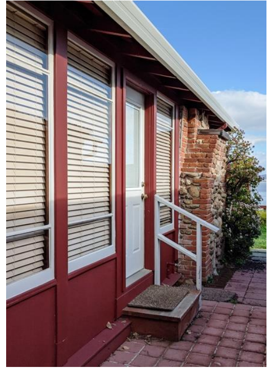
South Façade of Wrap-around Wing, incl. Front Door and Chimney. Viewed facing east. January 2020. (Photo by Leslie Dill)
