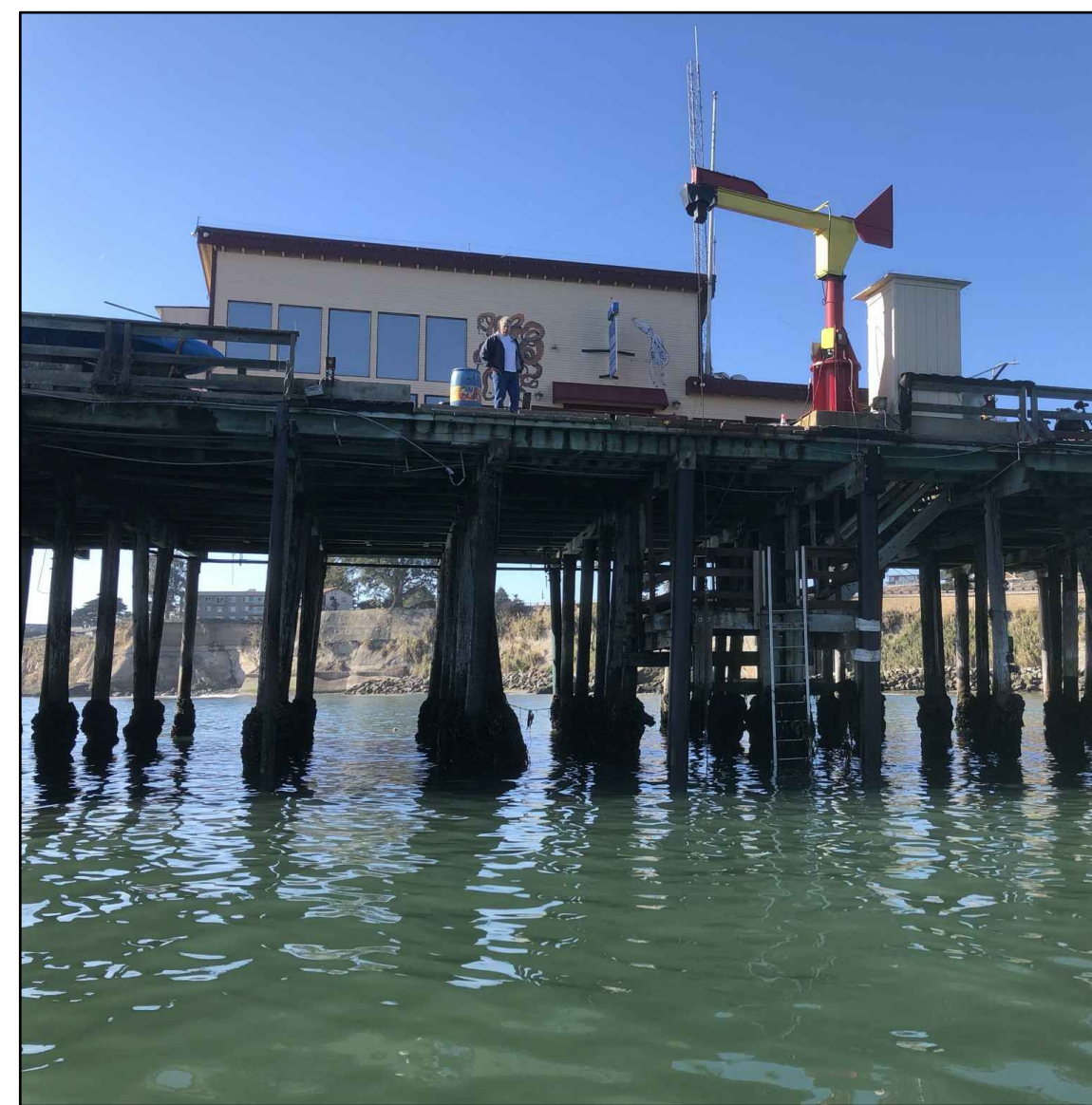
PHOTO 3 WHARF BELOW CRANE
