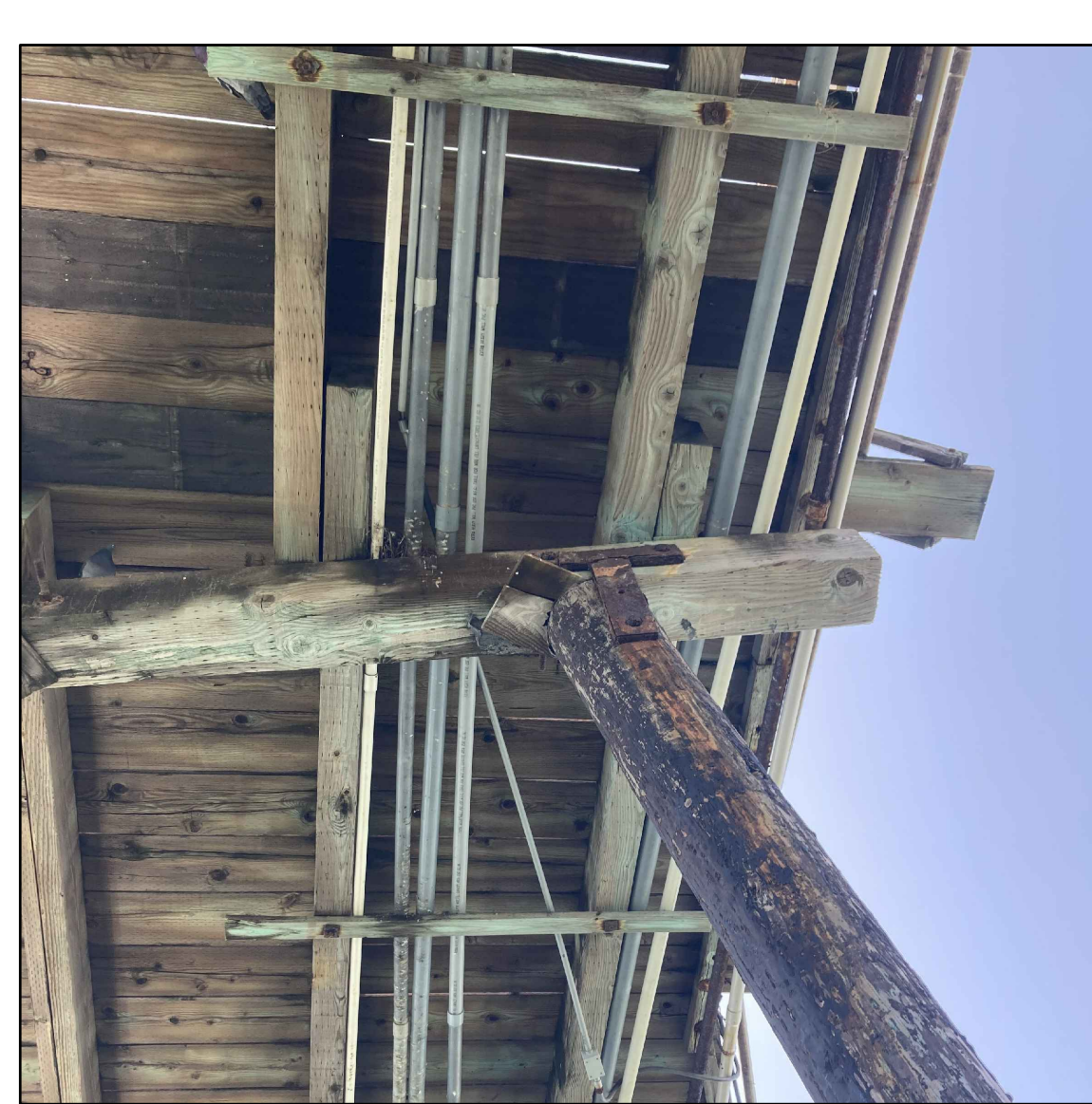
PHOTO 7 UTILITIES BELOW DECK
