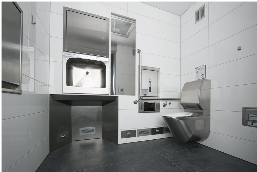
Figure 4. Exeloo restroom interior
