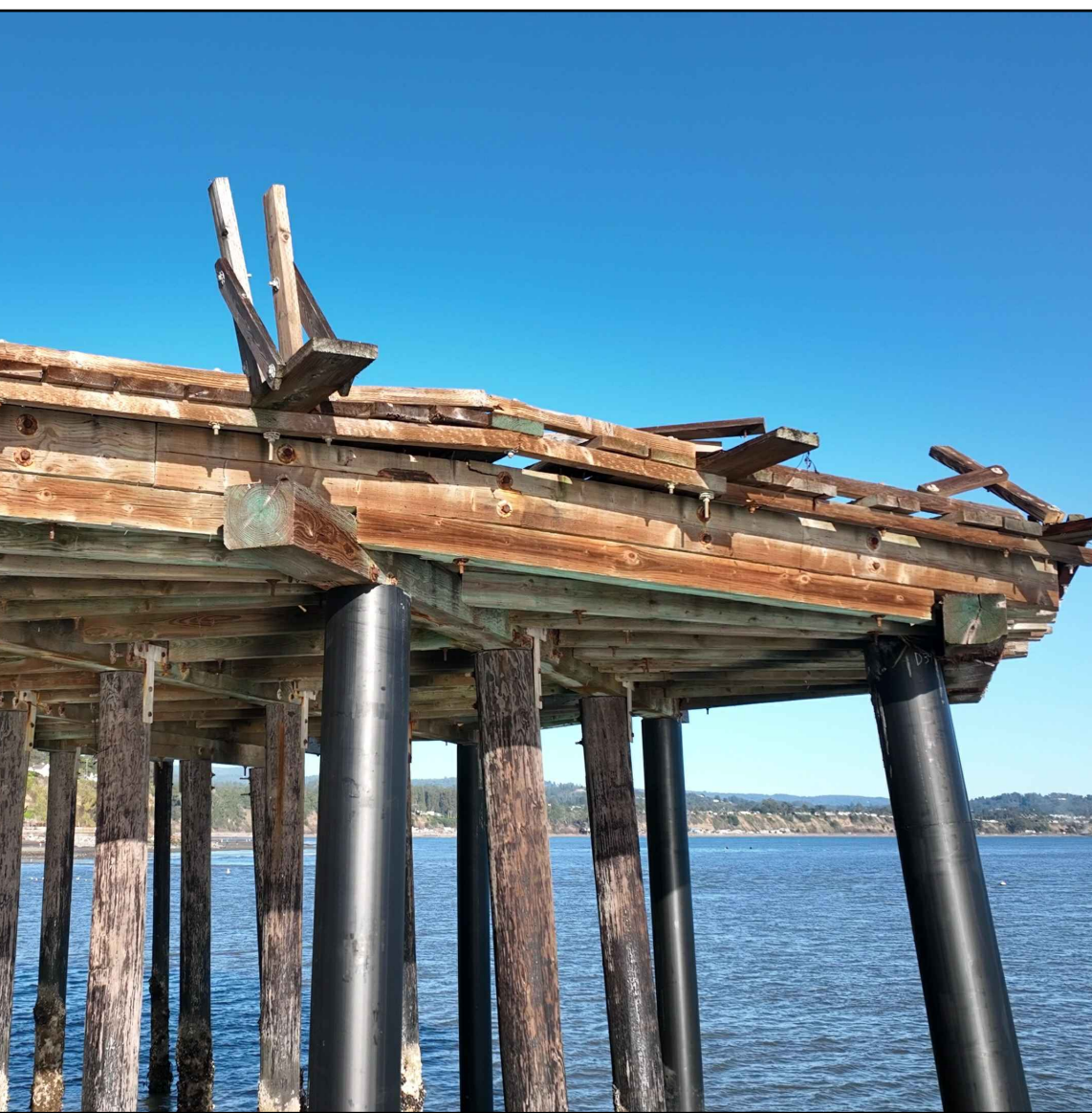
PHOTO 15 PILE CAPS AT WHARF HEAD
