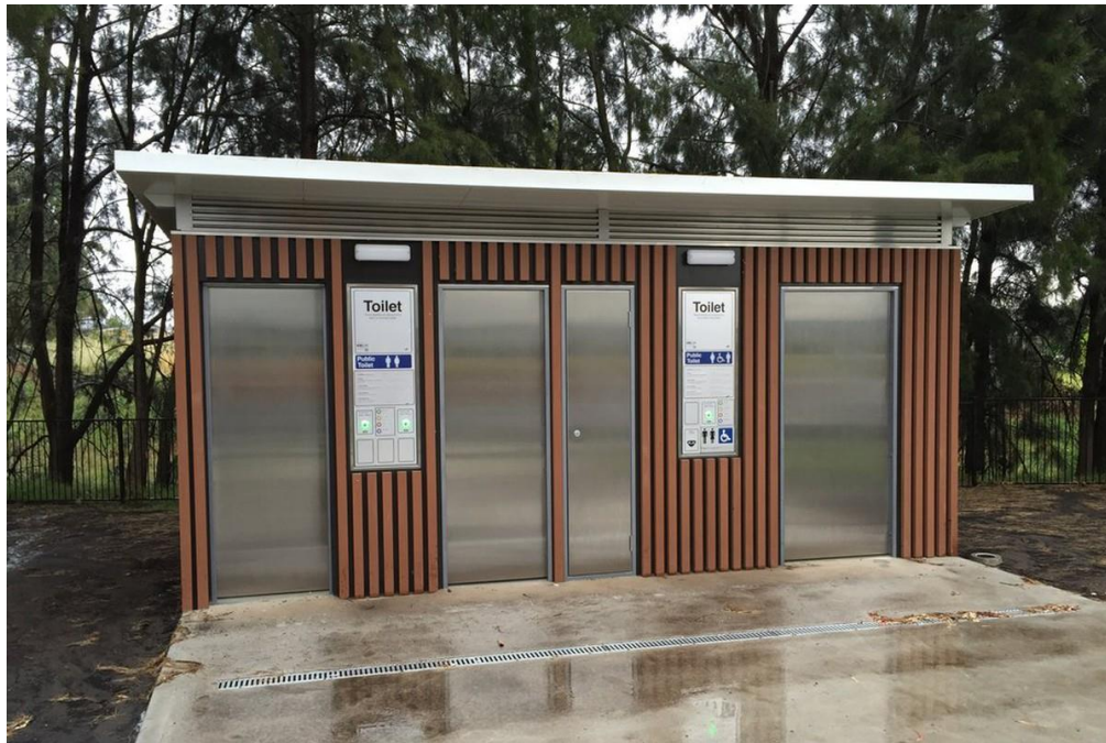
Figure 3. Exeloo triple cubicle restroom exterior
