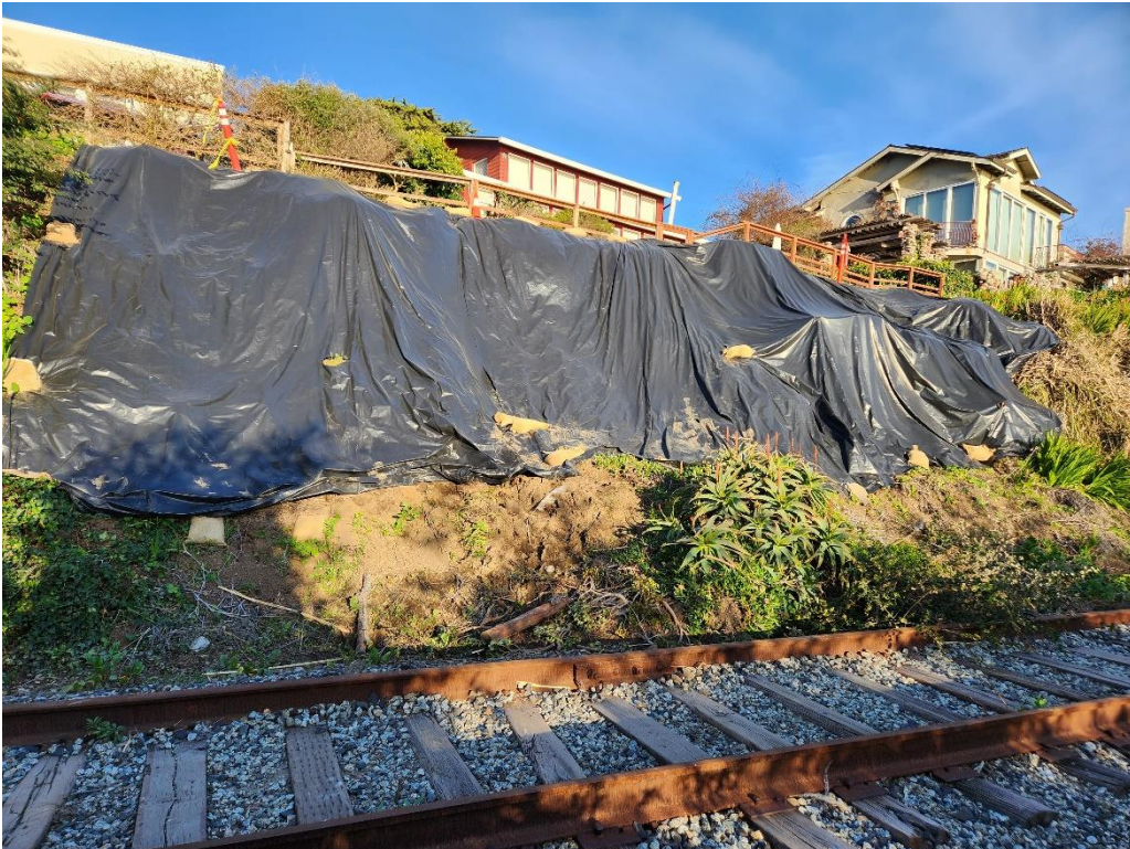
Figure 5. Slope failure adjacent to 1400 and 1410 Prospect Avenue
