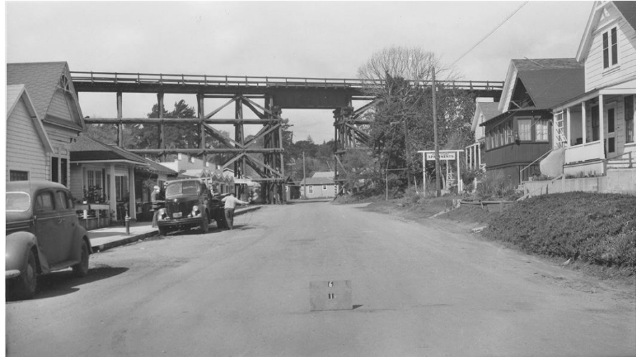
Historic trestle crossing Capitola Avenue
