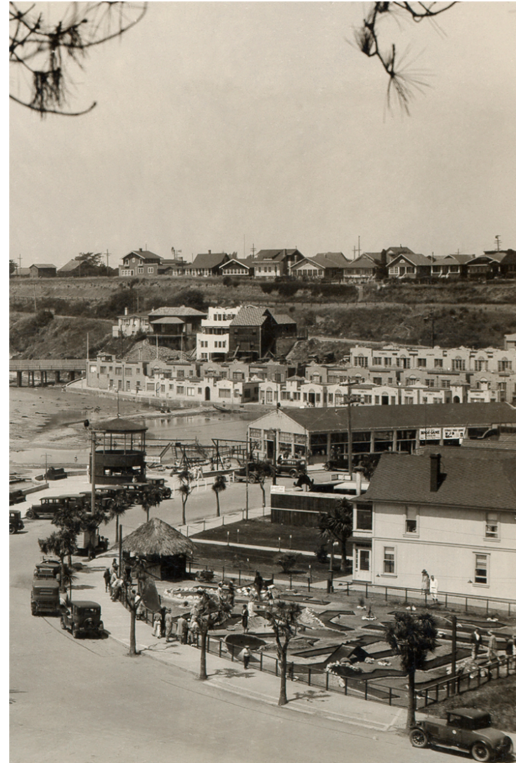
The Esplanade, Venetian, and Cliff Drive homes
