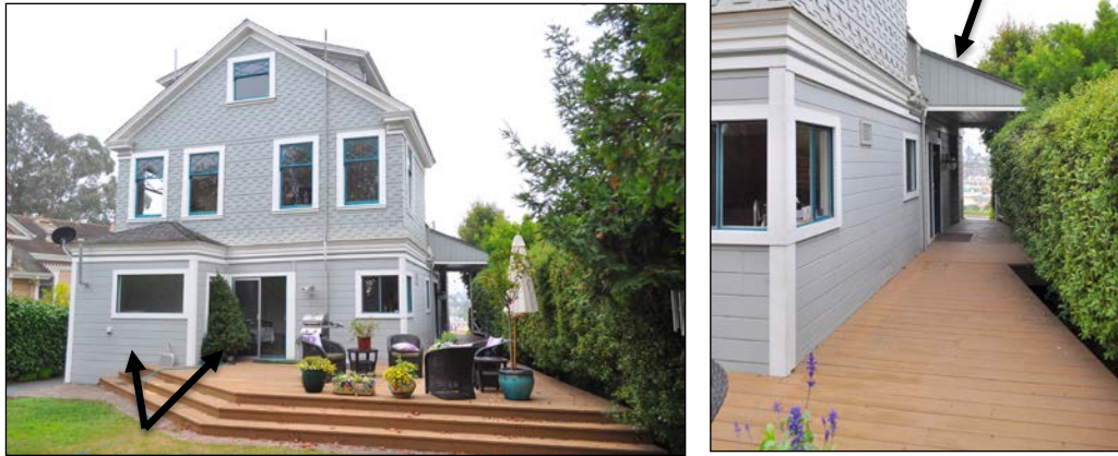
Figures 3 and 4. Left image shows the rear (east) elevation, with arrows indicating a rear addition and circa-1960s aluminum sliding glass doors. The upper-story wood sash windows are original. Right image details the north elevation, with modified entrance beneath the shed roof (arrow).
