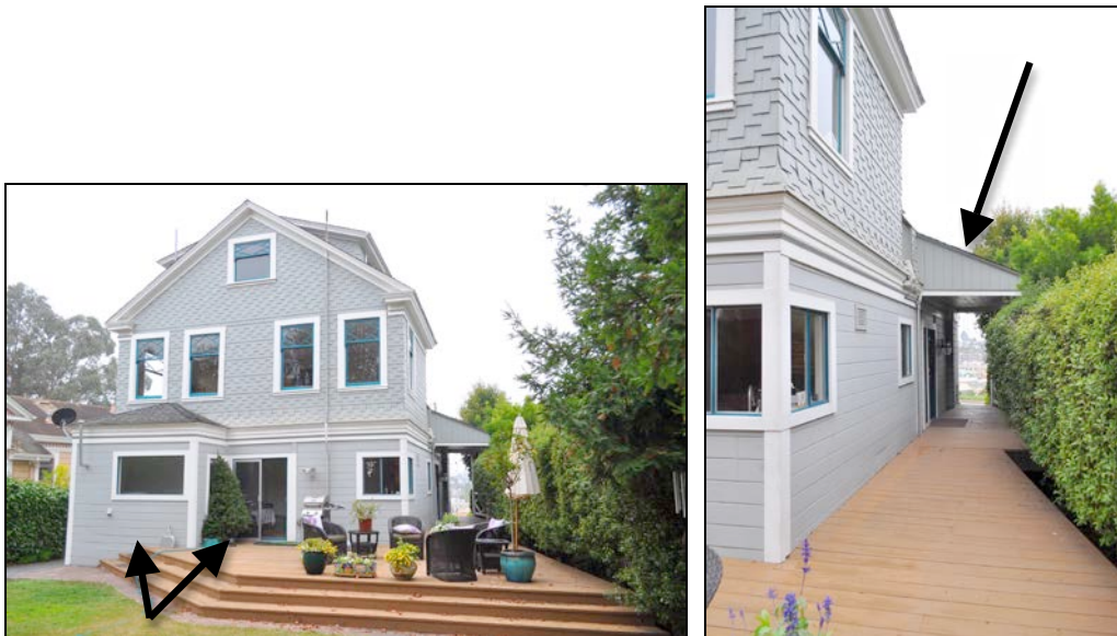
Figures 3 and 4. Left image shows the rear (east) elevation, with arrows indicating a rear addition and circa-1960s aluminum sliding glass doors. The upper-story wood sash windows are original. Right image details the north elevation, with modified entrance beneath the shed roof (arrow).
