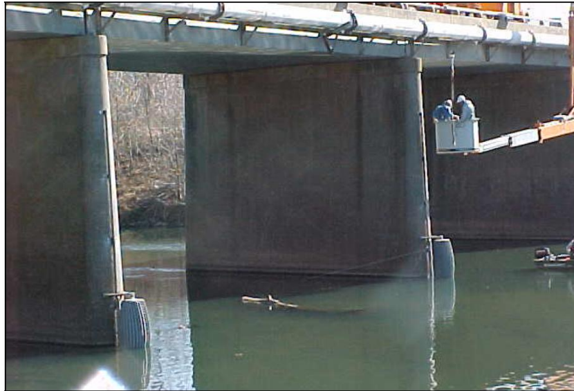
Figure 7. Photo of a debris sweeper being installed on bridge in Virginia
