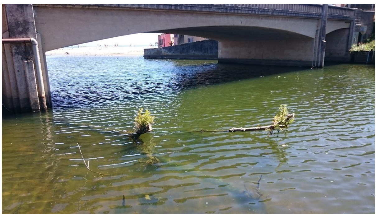
Figure 6. Photo, Looking Downstream, Stockton Avenue Bridge
