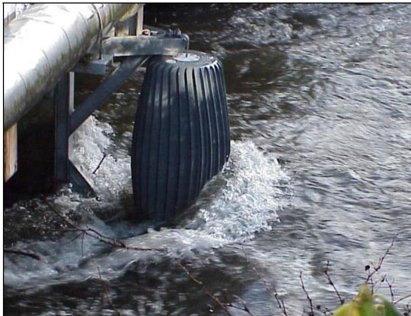
Figure 8. Photo close-up of a debris sweeper in Washington
