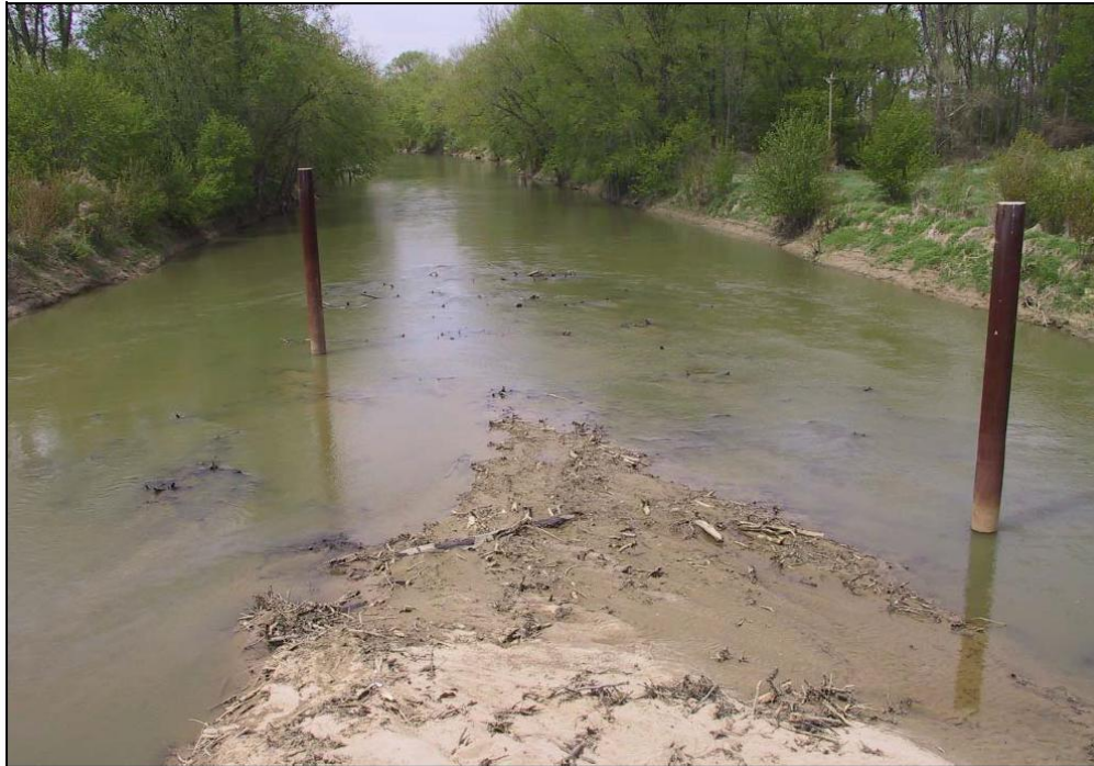
Figure 10. Photo of debris deflectors used in Indiana
