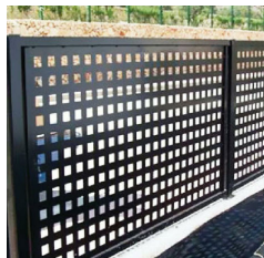
6C. PERFORATED METAL PANEL
