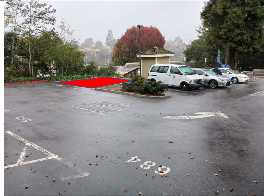
Location A – New Generator Site
