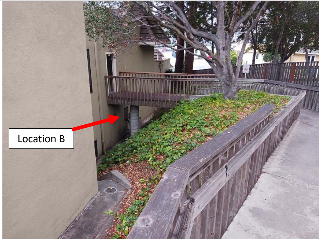
Location B – Electrical Room
