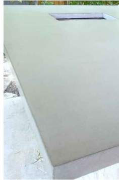
OUTDOOR KITCHEN CONCRETE COUNTER TOP
