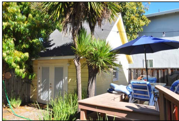
Figure 5. View of 1984 shed outbuilding located in the rear yard.
