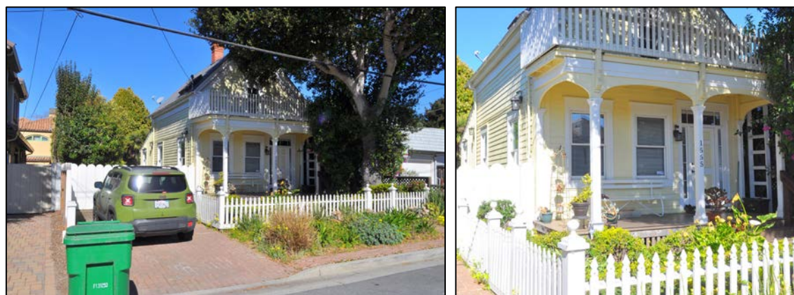
Figures 1 and 2. Left image shows the front (east) elevation, as viewed from the street. Right image details the front porch, which was replaced in the 1970s and the porch roof converted to a deck.
