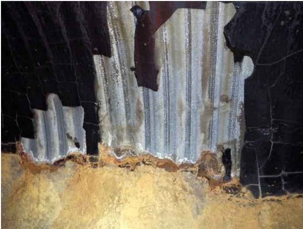
Photo 25. Station 2+96; typical section of coating failure, corrugated metal in good condition.
