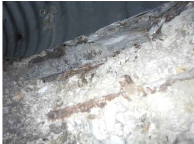
Photo 10. Station 0+85; exposed reinforcement at lateral.
