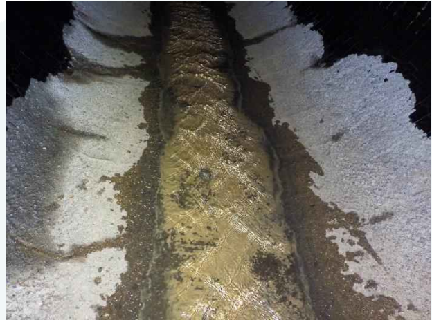
Photo 16. Station 2+00; grout along bottom of pipe.
