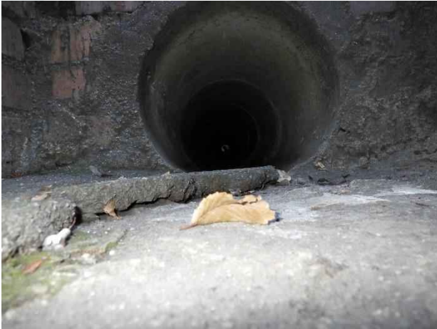
Photo 11. Station 2+67; storm drain inlet in good condition.
