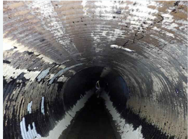
Photo 33. Station 0+95; coating failure along pipe, corrugated metal was in good condition.
