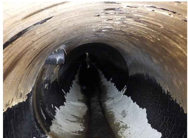
Photo 24. Station 0+80; coating discoloration from 9:00 to 3:00.
