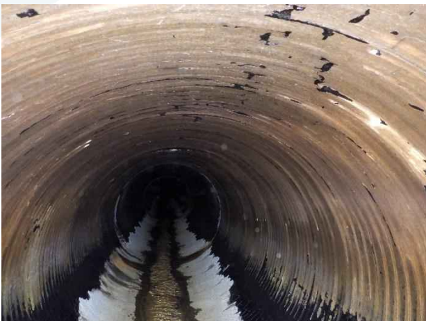
Photo 15. Station 2+00; coating discoloration from 8:00 to 4:00 of pipe.
