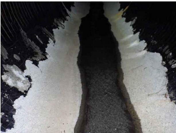
Photo 23. Station 0+80; concrete grout along the bottom of the pipe; typical for segment 1.
