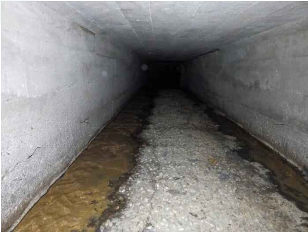
Photo 5. Station 0+54; outfall box culvert in good condition.
