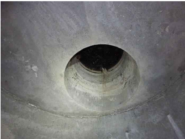
Photo 36. Station 1+25; concrete manhole was in good condition.
