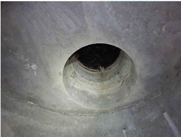
Photo 34. Station 1+25; concrete manhole was in good condition.
