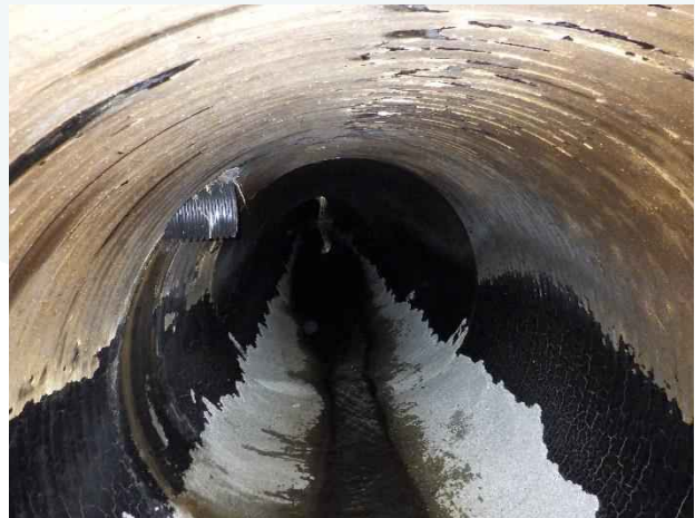
Photo 22. Station 0+80; coating discoloration from 9:00 to 3:00.
