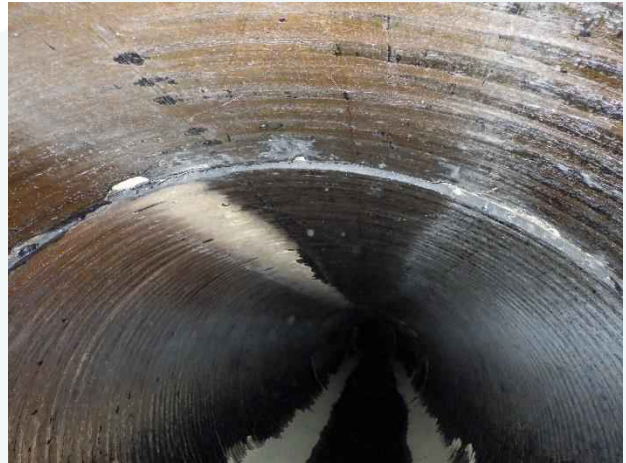
Photo 33. Station 0+46; coating uneven at joint.
