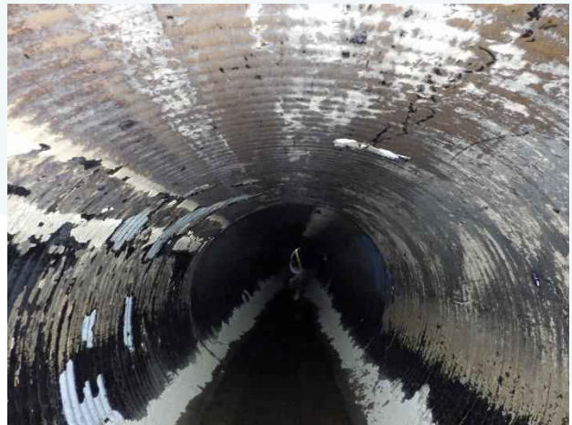
Photo 35. Station 0+95; coating failure along pipe, corrugated metal was in good condition.
