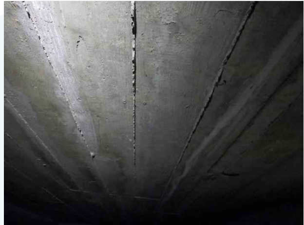
Photo 6. Station 1+00; box culvert ceiling in good condition.
