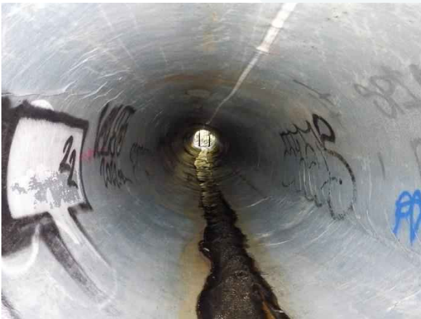
Photo 42. Station 0+70; CIPP liner deformed (squished) but in good condition.
