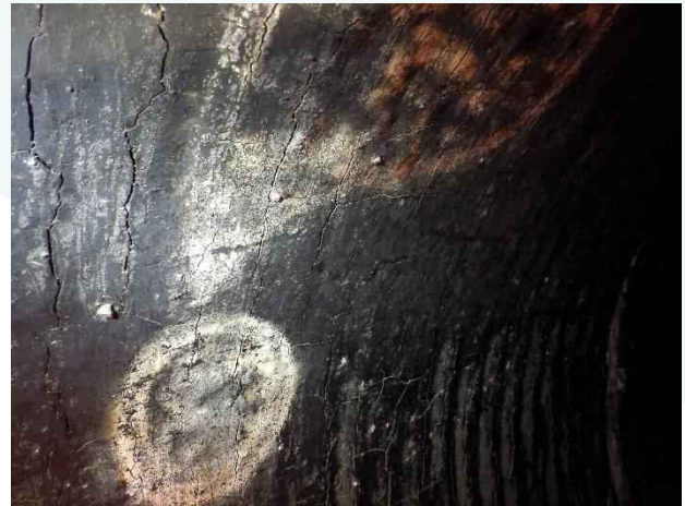
Photo 22. Station 0+00; typical craze pattern cracking of coal tar coating.
