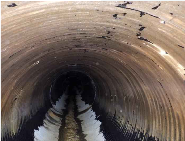
Photo 17. Station 2+00; coating discoloration from 8:00 to 4:00 of pipe.
