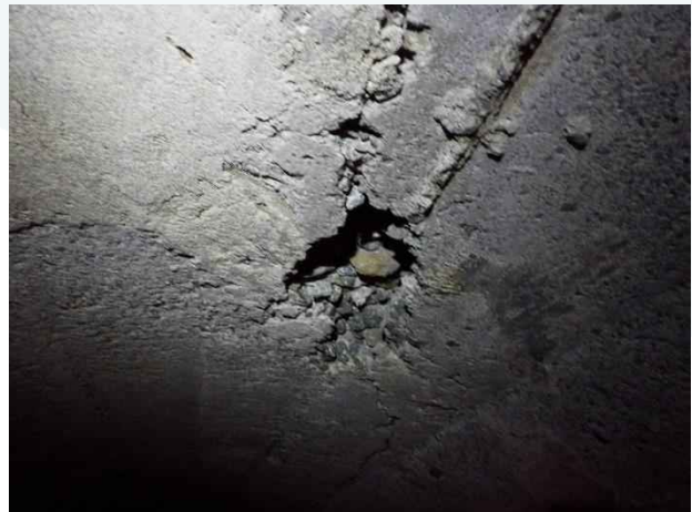
Photo 39. Station 0+14; concrete spalling on arch pipe.
