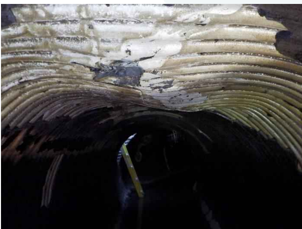
Photo 17. Station 3+54; deformed bulge defect on the crown of the pipe.
