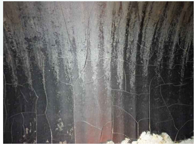
Photo 12. Station 0+07; craze pattern cracking of coating.
