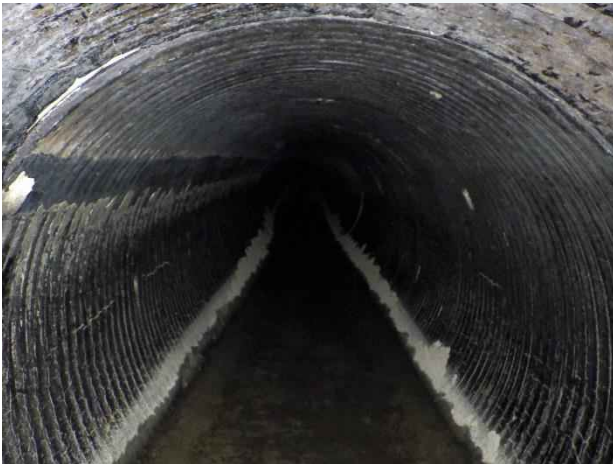
Photo 21. Station 0+00; signs of coal tar deterioration along pipe.
