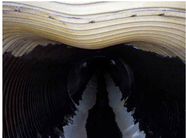
Photo 24. Station 2+05; bulge deformation defect on the crown of the pipe.
