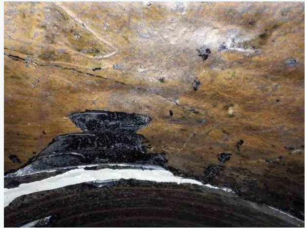
Photo 29. Station 0+84; deteriorated coating on the crown of the pipe.
