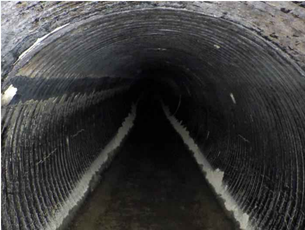
Photo 19. Station 0+00; signs of coal tar deterioration along pipe.
