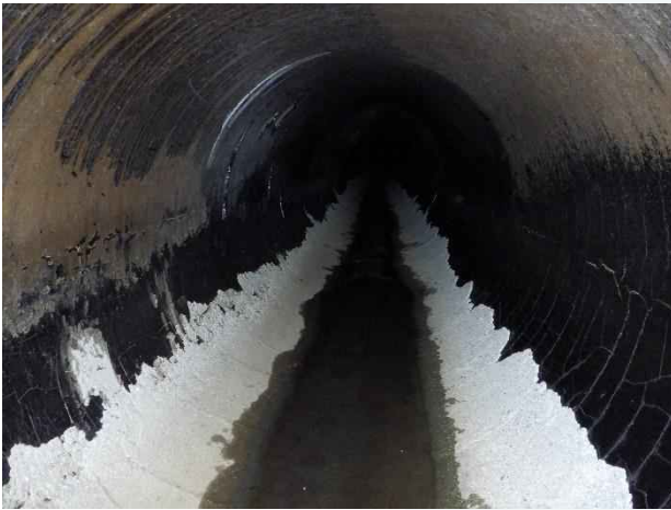
Photo 28. Station 0+00; signs of coal tar deterioration and discoloration along pipe.
