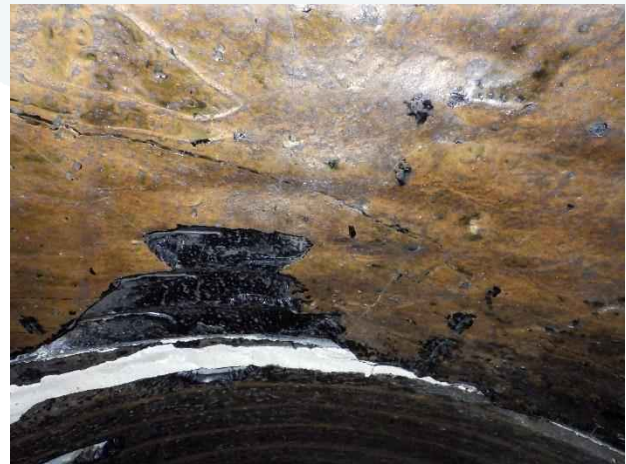
Photo 31. Station 0+84; deteriorated coating on the crown of the pipe.
