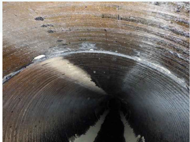
Photo 31. Station 0+46; coating uneven at joint.
