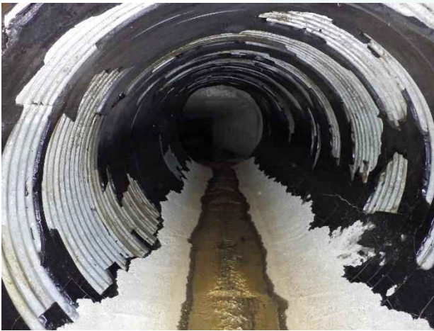
Photo 11. Station 0+07; coal tar coating failure along pipe.
