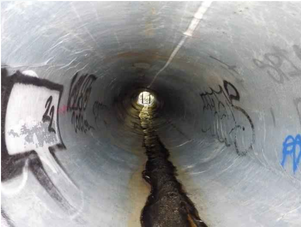
Photo 40. Station 0+70; CIPP liner deformed (squished) but in good condition.
