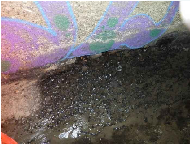
Photo 36. Station 0+14; minor concrete void along the bottom of the arch pipe.
