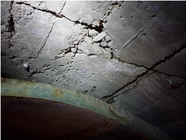
Photo 40. Station 0+70; large cracks and exposed aggregate on arch pipe.
