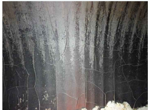
Photo 14. Station 0+07; craze pattern cracking of coating.
