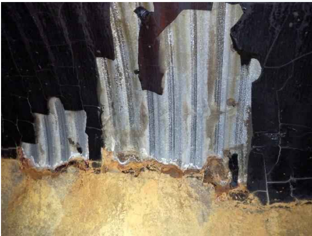
Photo 27. Station 2+96; typical section of coating failure, corrugated metal in good condition.
