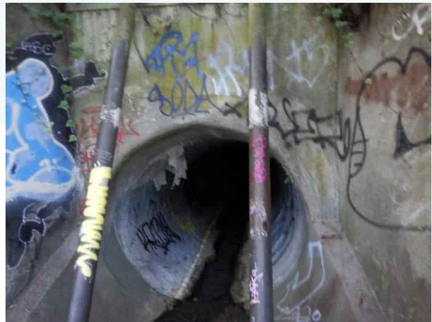
Photo 43. Noble Gulch; bar screen entrance in good condition.
