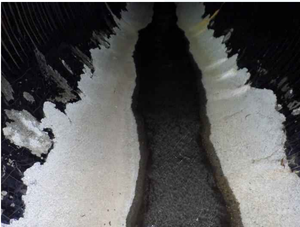
Photo 21. Station 0+80; concrete grout along the bottom of the pipe; typical for segment 1.
