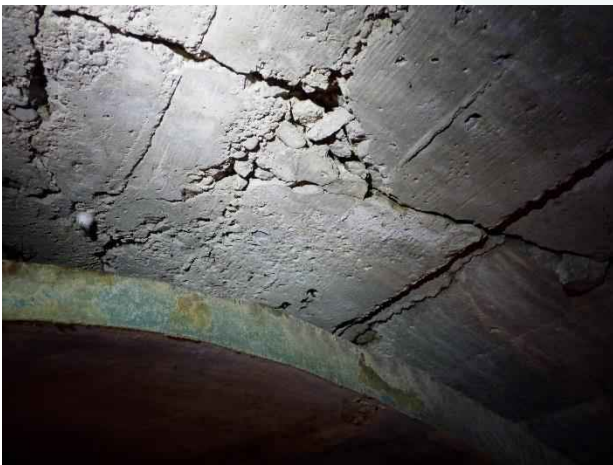
Photo 38. Station 0+70; large cracks and exposed aggregate on arch pipe.
