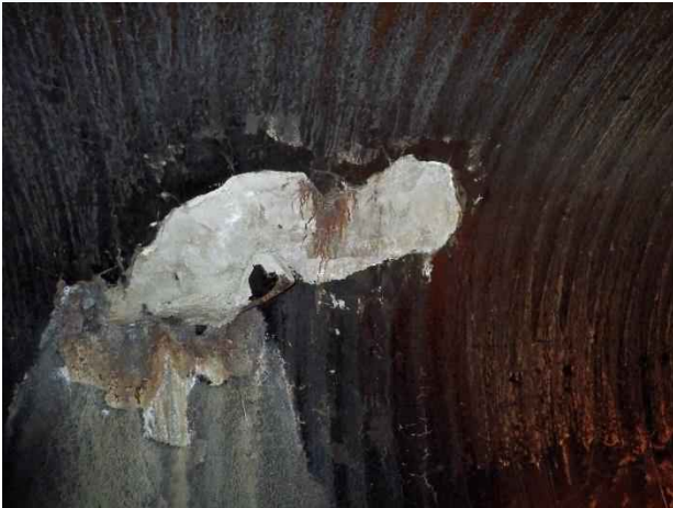
Photo 32. Station 0+46; repair patch at the 3:00 position.
