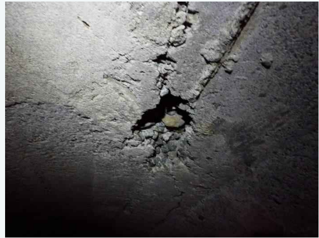
Photo 37. Station 0+14; concrete spalling on arch pipe.
