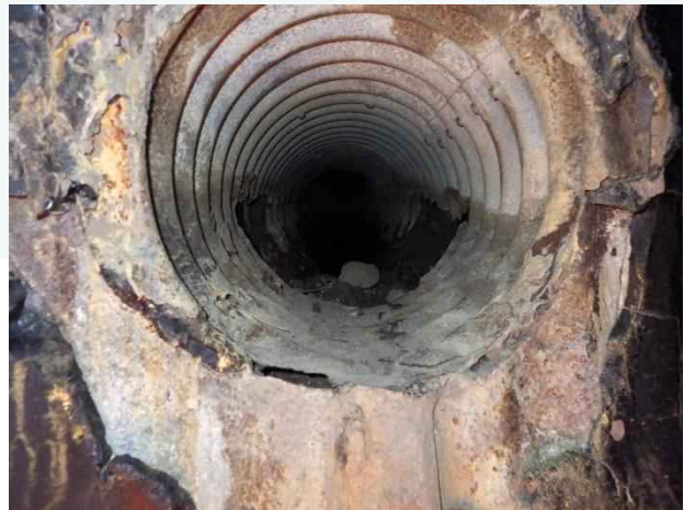
Photo 18. Station 2+80; lateral with minor corrosion at pipe intersection.
