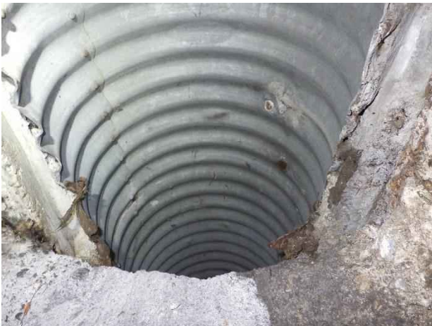
Photo 9. Station 0+85; lateral in box culvert ceiling.
