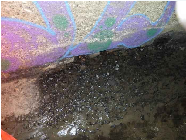
Photo 38. Station 0+14; minor concrete void along the bottom of the arch pipe.
