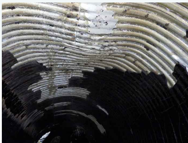
Photo 18. Station 3+54; signs of minor corrosion on deformed bulge.
