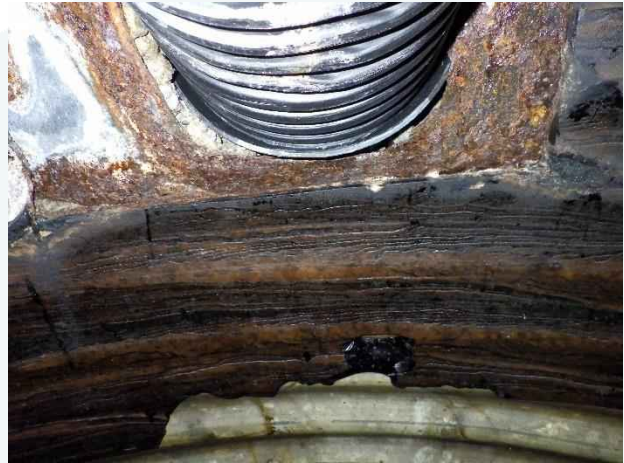
Photo 26. Station 3+84; minor corrosion of metal at lateral break in site.
