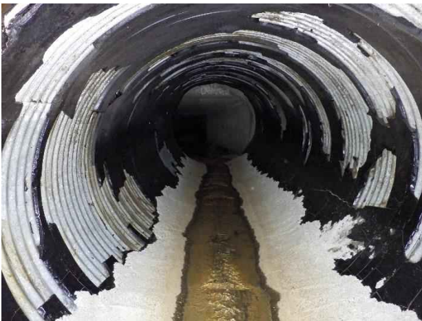
Photo 13. Station 0+07; coal tar coating failure along pipe.
