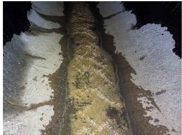
Photo 14. Station 2+00; grout along bottom of pipe.
