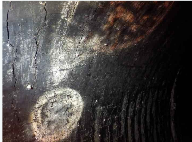
Photo 20. Station 0+00; typical craze pattern cracking of coal tar coating.
