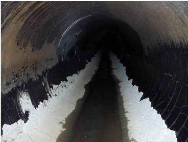
Photo 30. Station 0+00; signs of coal tar deterioration and discoloration along pipe.
