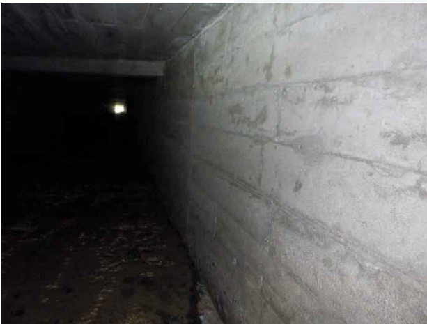
Photo 7. Station 1+00; box culvert wall in good condition.
