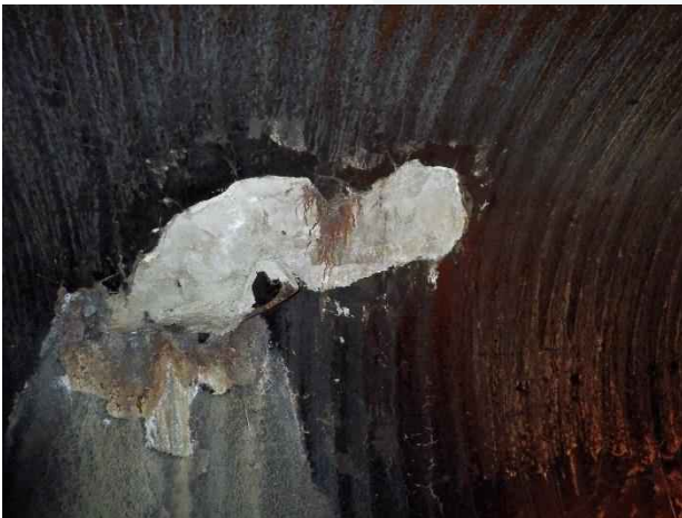
Photo 34. Station 0+46; repair patch at the 3:00 position.
