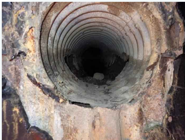
Photo 16. Station 2+80; lateral with minor corrosion at pipe intersection.
