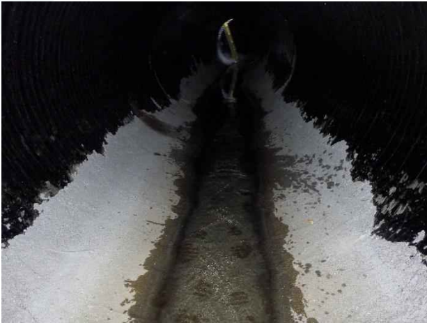
Photo 32. Station 0+46; concrete grout along the bottom of the pipe in good condition.
