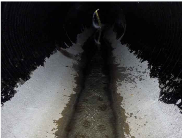
Photo 30. Station 0+46; concrete grout along the bottom of the pipe in good condition.
