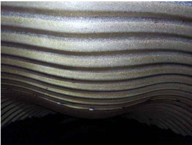
Photo 23. Station 1+80; bulge deformation defect on the crown of the pipe.
