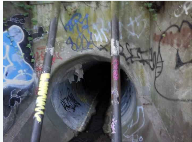
Photo 41. Noble Gulch; bar screen entrance in good condition.
