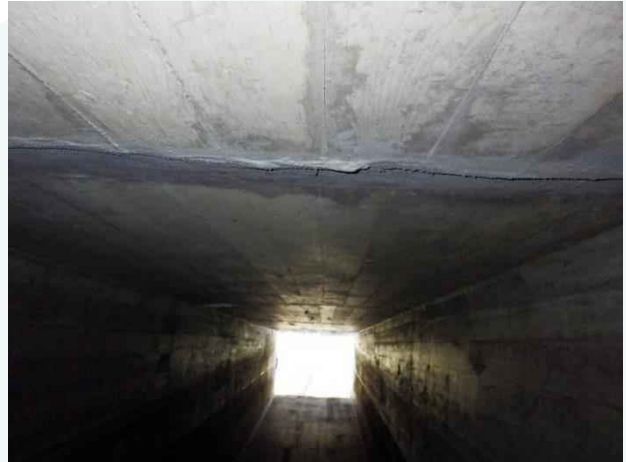
Photo 12. Station 3+53; mortared joint in good condition.
