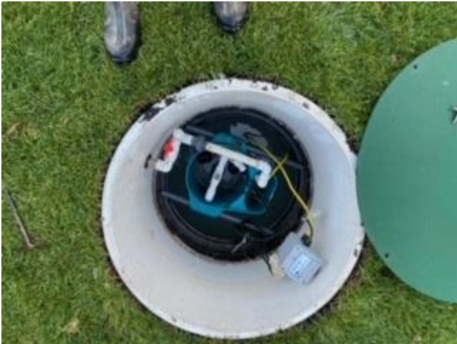
Figure 3: New Replaement Floats in STEP Tank
