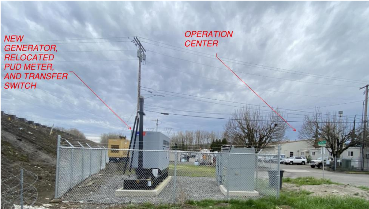
Generator Installation on Polk Street
