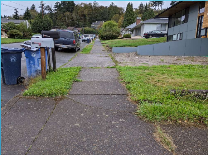
NW 19 TH AVE, LOOKING WEST TO NW BENTON ST
