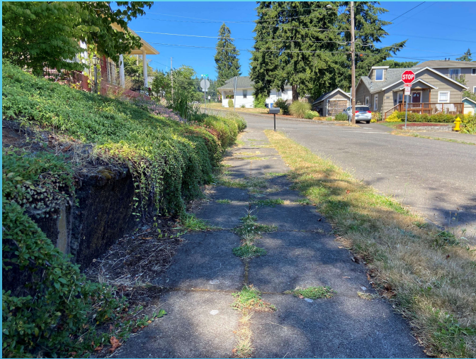
NW BENTON ST, LOOKING NORTH TO NW 16 TH AVE
