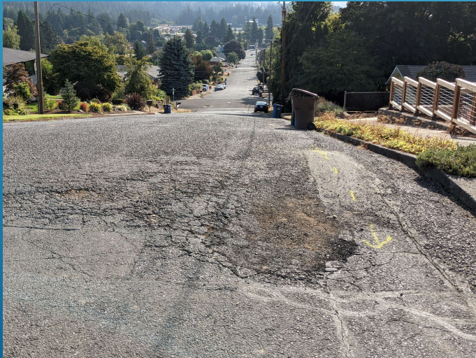
NW 21 ST AVE, LOOKING EAST TO NW BENTON ST
