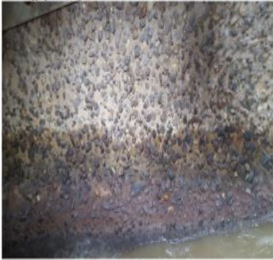
Figures 1-2: Damaged concrete in Headworks
