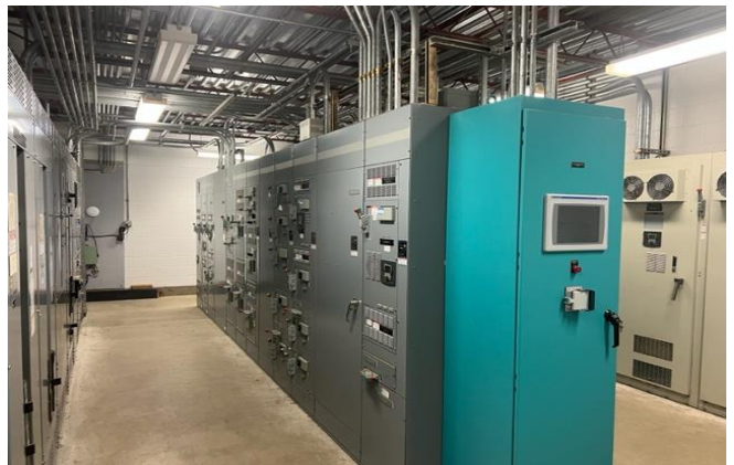
Fig. 6 Electrical Room HVAC upgrades
