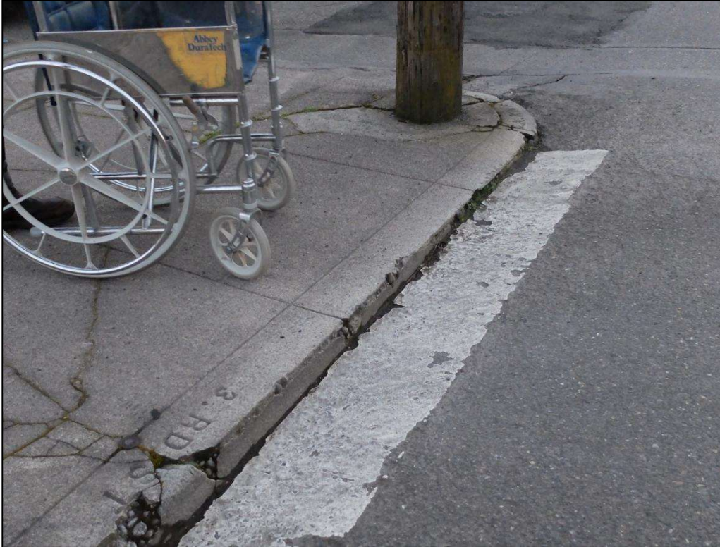
Figure 3: Example of full height curb that is a barrier to the disabled
