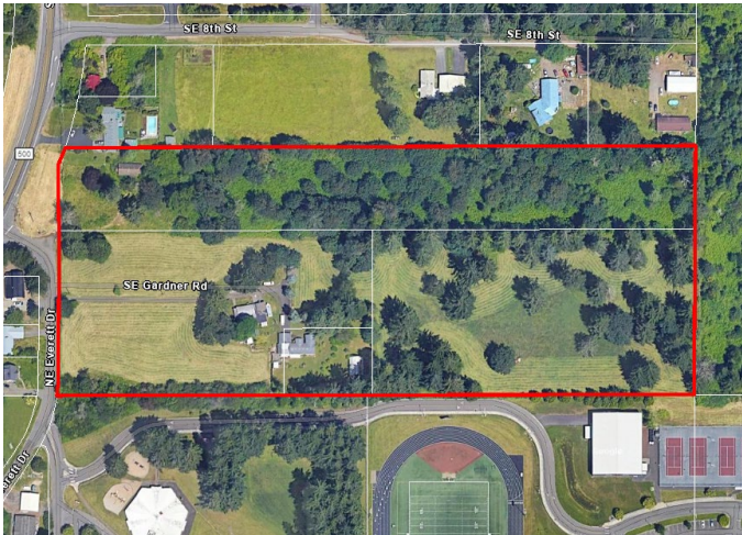
3. Camas Woods-West Portion
