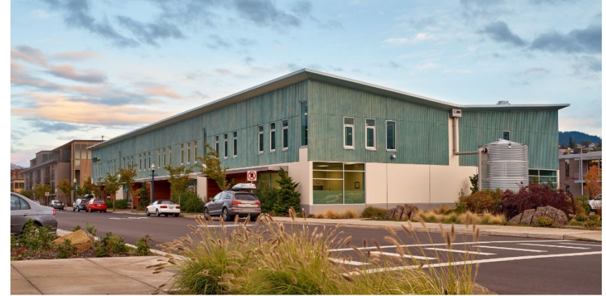
At the LEED Silver Halyard Building in Hood River, OR, rooftop equipment is screened from the street, parking is located behind the building, and a stormwater cistern collects runoff.
