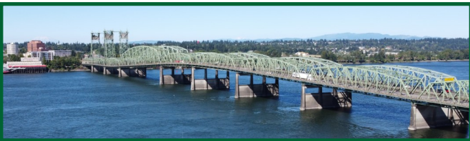
108-year-old I-5 Bridge.
