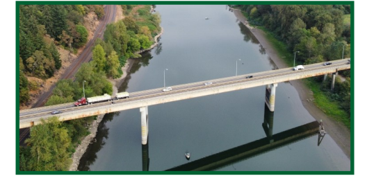
60-year-old West Camas Slough Bridge.
