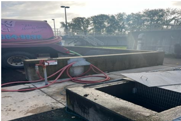
Fig 5 Septage Receiving Station
