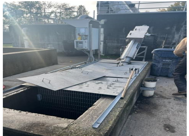
Fig. 8 Septage Receiving Station
