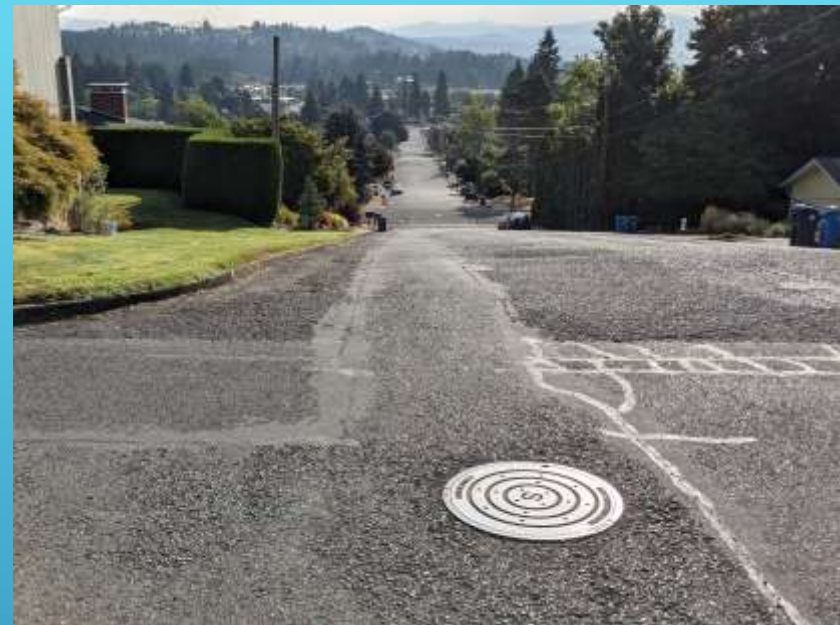
NW 21 ST AVE AT NW COUCH ST, LOOKING EAST
