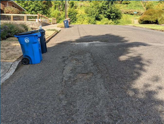
NW 21 ST AVE. LOOKING WEST
