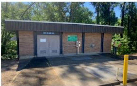
Fig.5: Front of Pump Station
