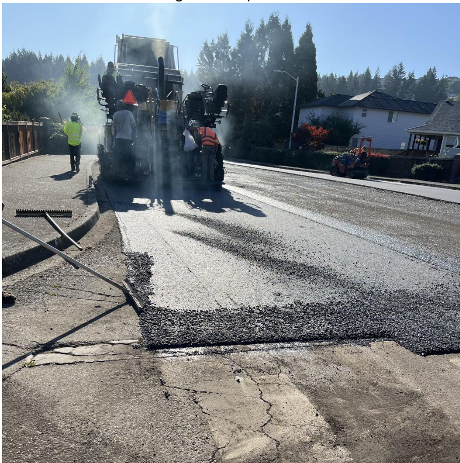
New Wearing Surface placed in Two Lifts
