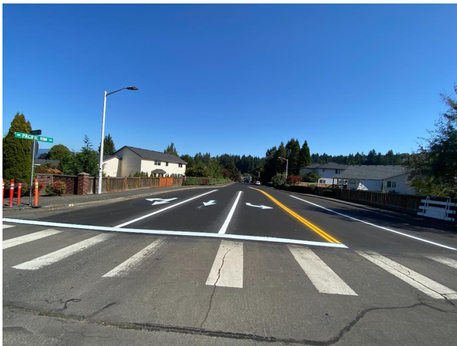
New Wearing Surface placed in Two Lifts
