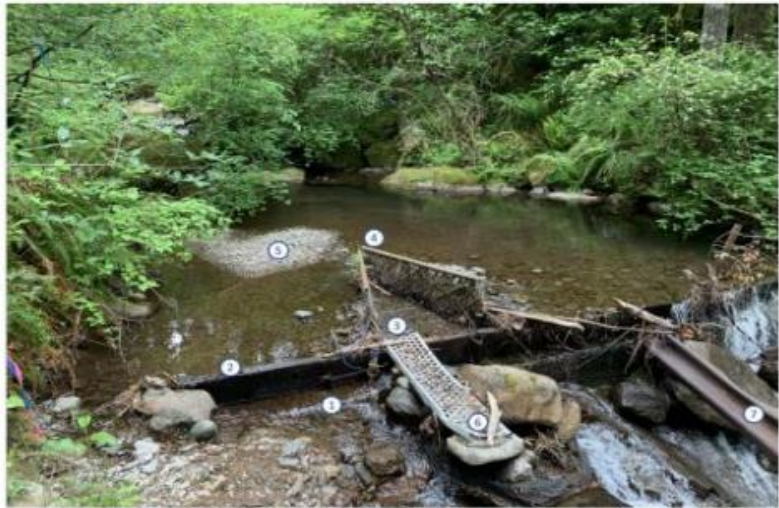
Figure 1: Photo of existing dam and intake structure from downstream of dam looking upstream
