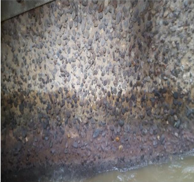
Figures 1-2: Damaged concrete in Headworks
