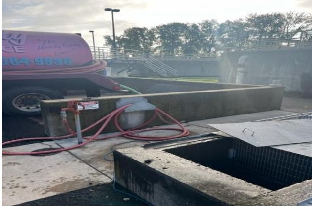
Fig 7 Septage Receiving Station
