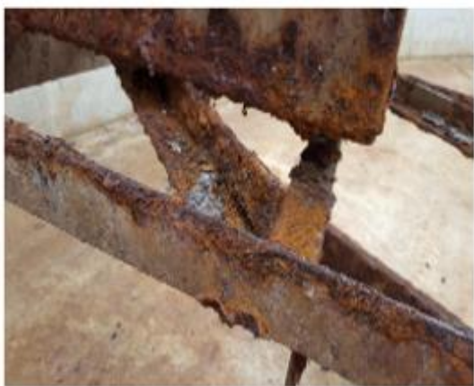
Figures 3-5: Corroded Metal in Primary Clarifier Basin
