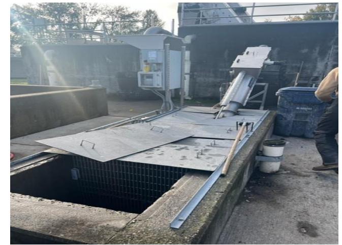
Fig. 10 Septage Receiving Station
