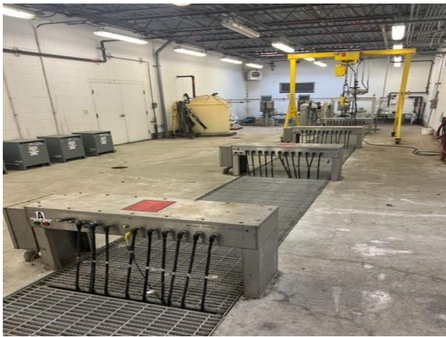
Fig. 9 Ultraviolet (UV) Bank
