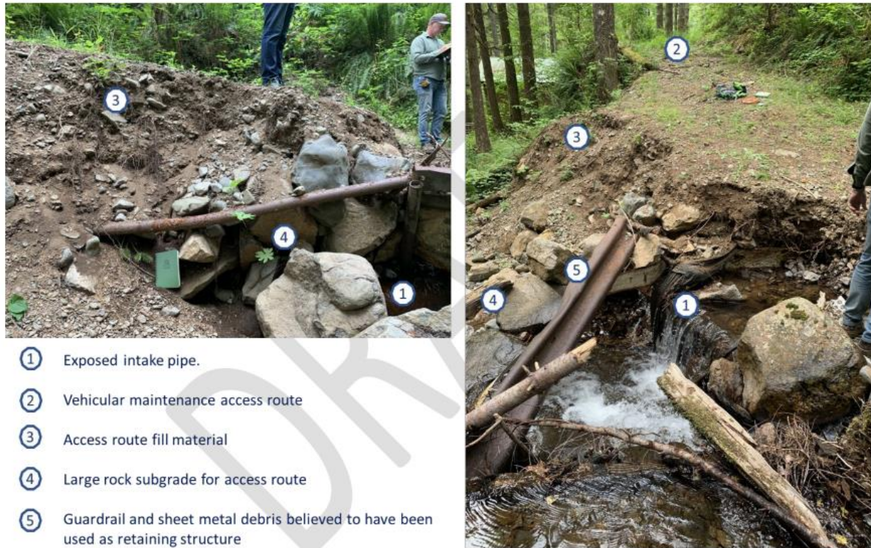
Figure 3: Existing bank erosion along right bank of Boulder Creek looking downstream in intake structure.
