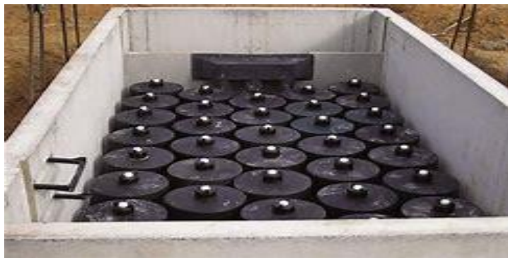
Figure 2: Storm filter vaults example
