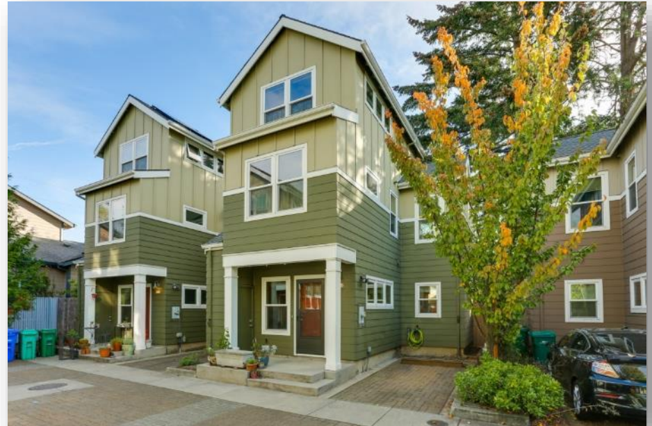
Recent home purchased through Proud Ground, Portland, From https://proudground.org/
