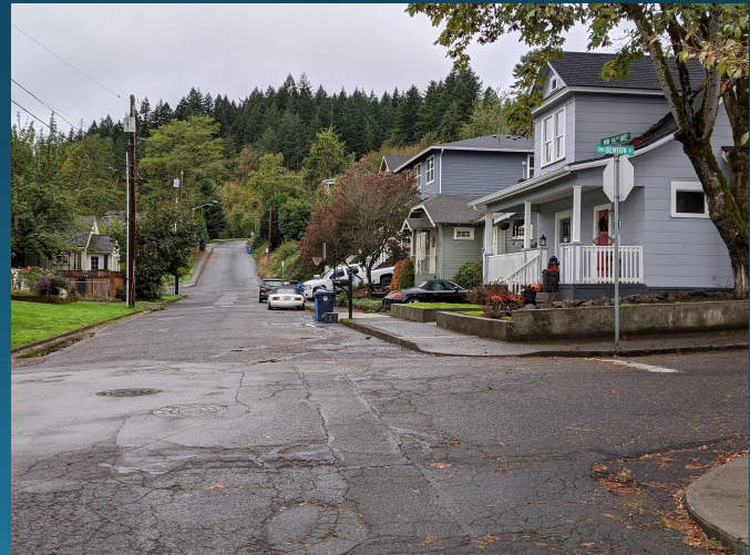
NW 14 TH AVE. AT NW BENTON ST. LOOKING WEST
