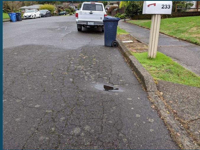
NW 19 TH AVE. LOOKING WEST TOWARDS NW BENTON ST.
