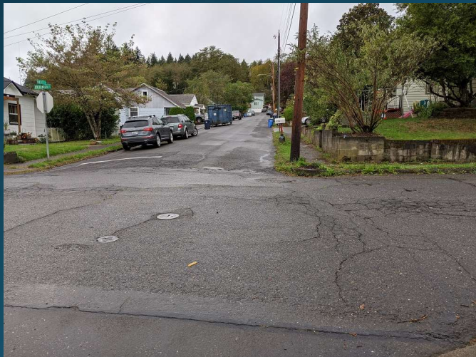
NW BENTON ST. AT NW 17 TH AVE. LOOKING WEST
