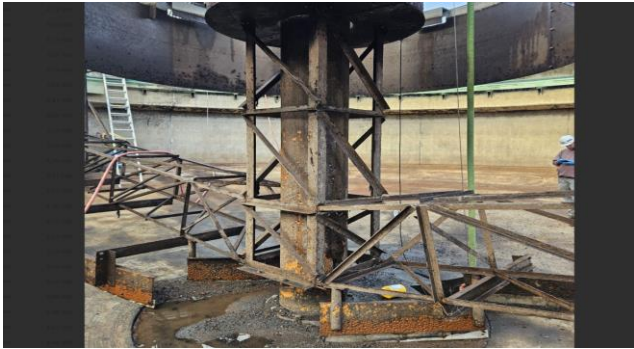
Figure 2-4: Clarifier Arm Damage
