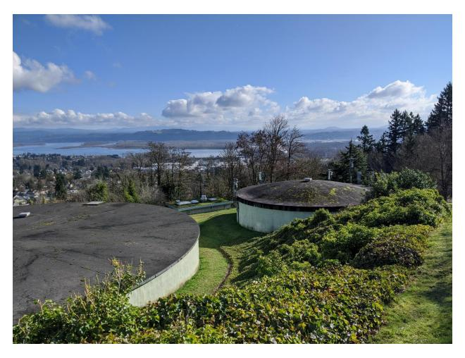
Lower Prune Hill Reservoir Site: Existing 500,000-gallon tank (right side) and booster station (center).
