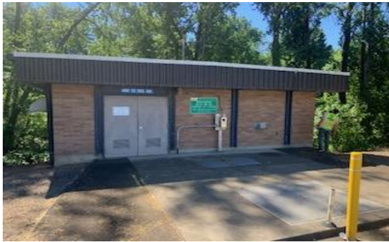
Fig.5: Front of Pump Station
