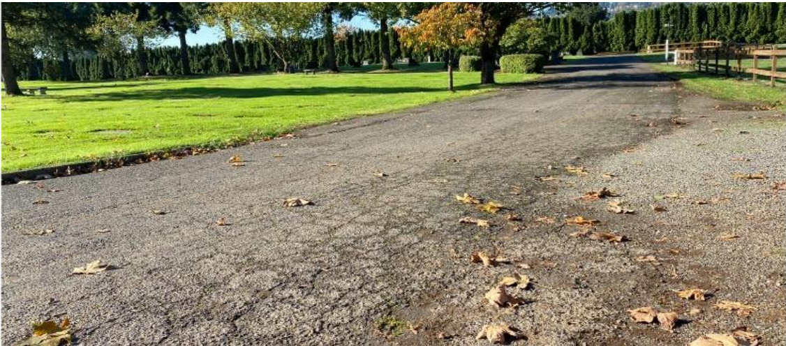
Pavement Condition Sample
