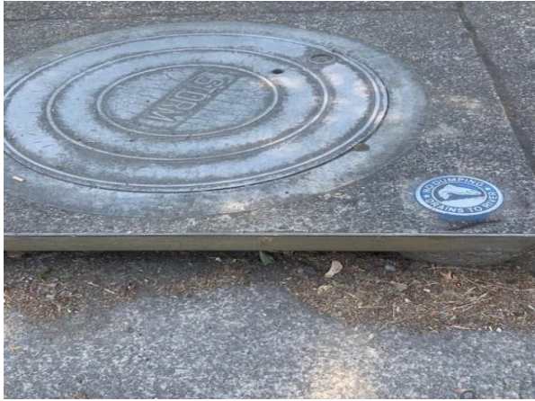
Figure 1: Curb inlet with Camas medallion
