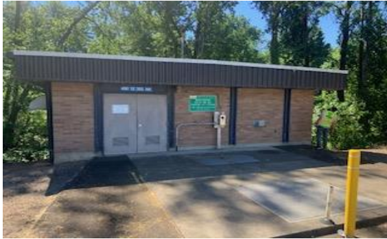
Fig.5: Front of Pump Station
