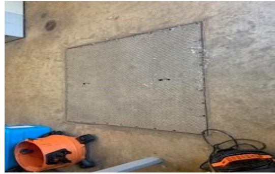
Fig 4: Substandard Hatch for Pump Access
