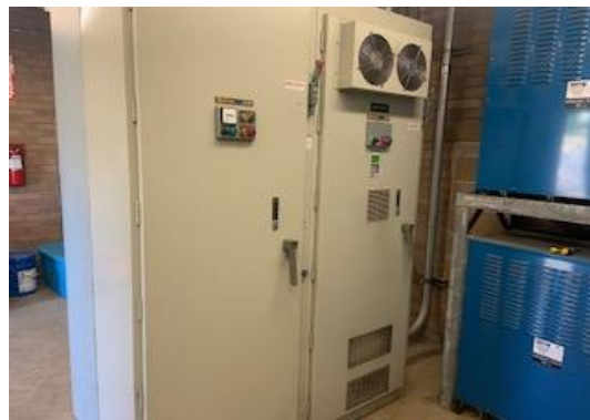
Fig 2: Variable Frequency Drive Panel
